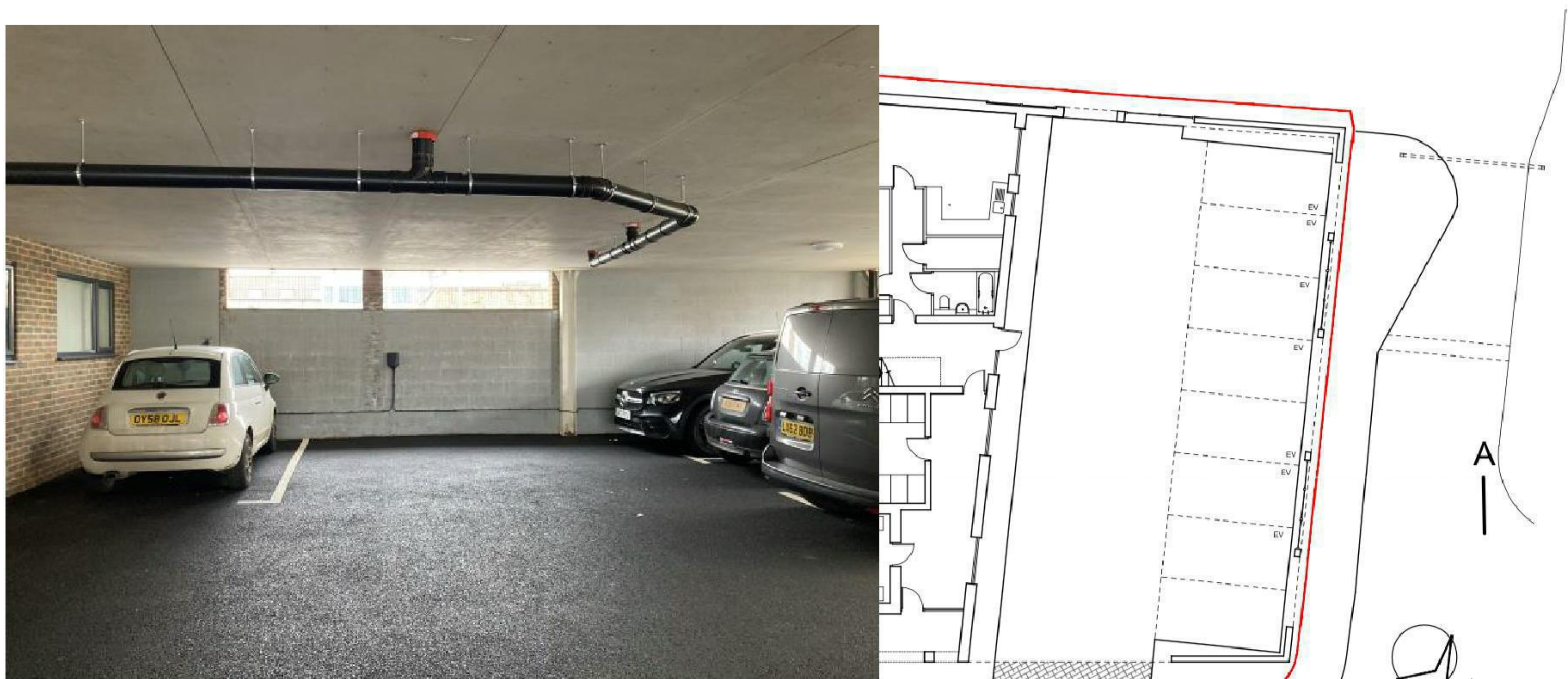
Unauthorised 9 th space; EV point for potential 10 th space; original approved plan
