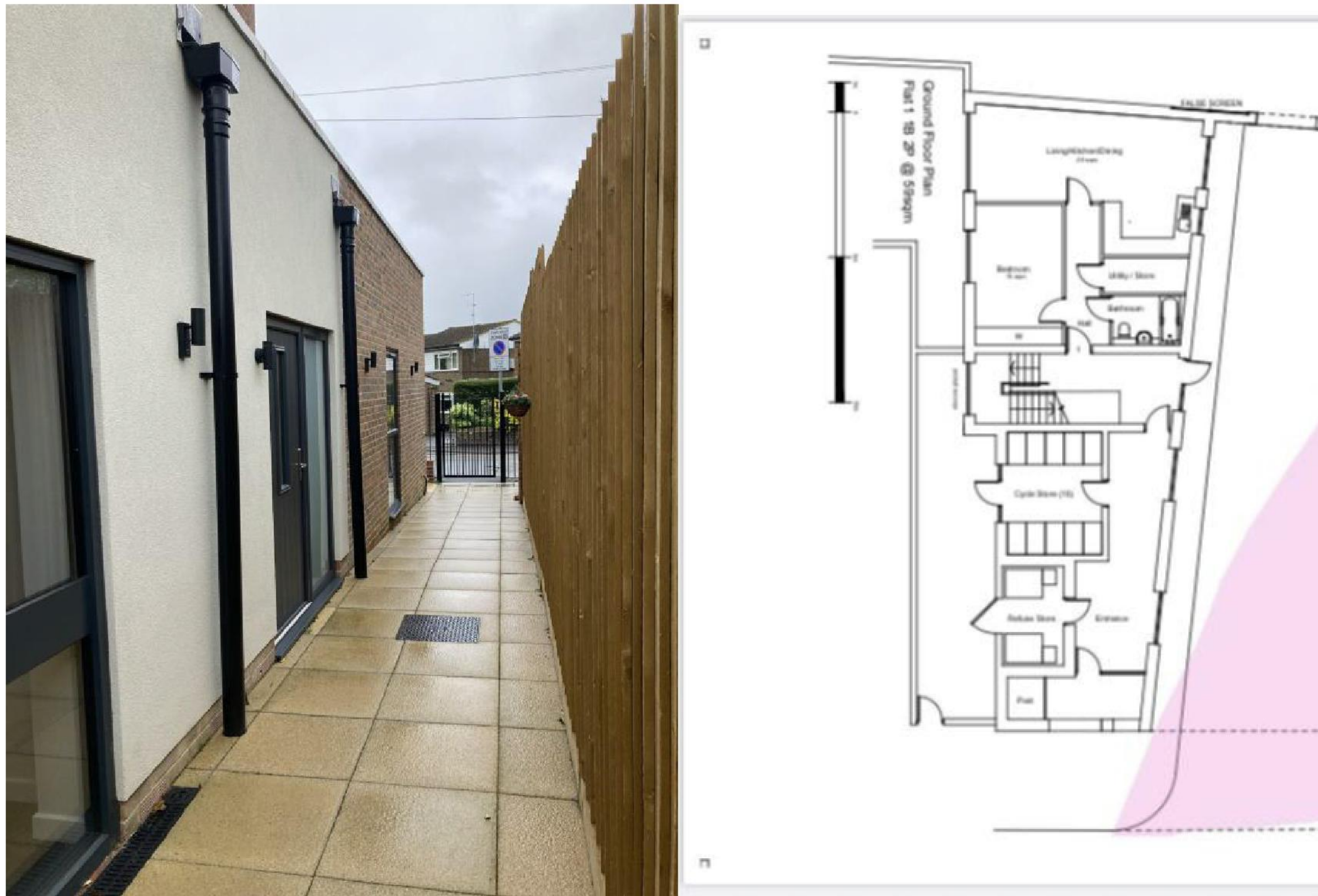
The walkway has been cut back to maximise the floor space for a potential 10 th flat
