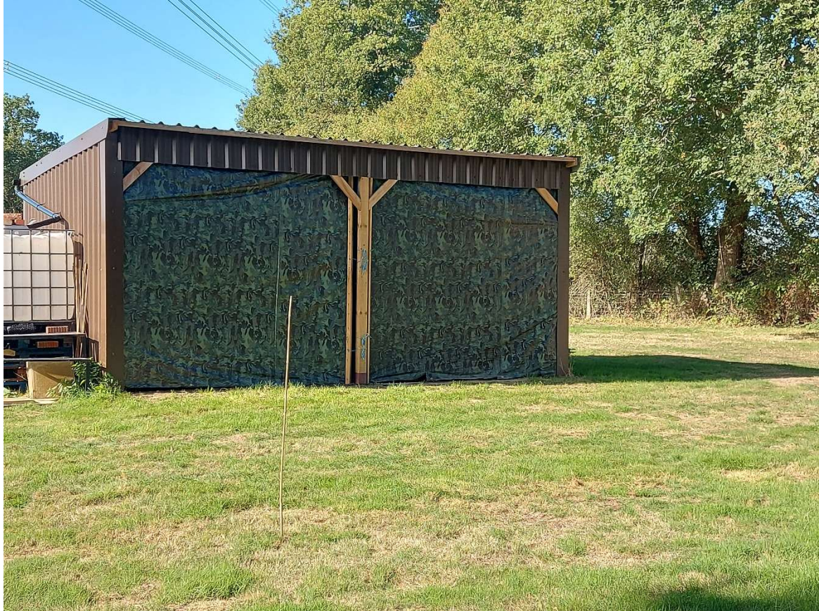
Existing machinery shed
