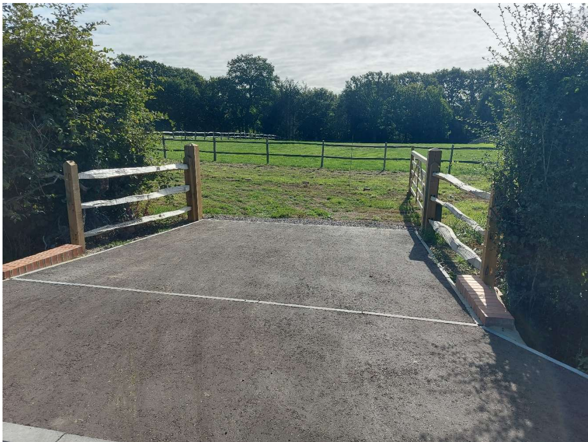
The recently constructed site entrance
