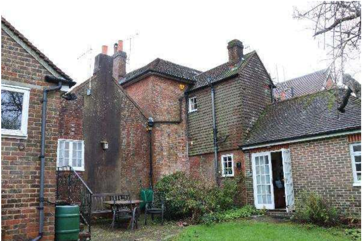
5. Rear Elevation General view
