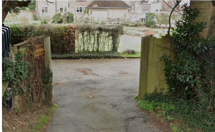
Figure 5 – Photograph of the London Lane boundary showing closeboard fencing attached to the structure of the building (source Google Street Map 2021)
