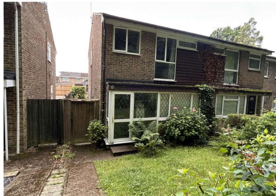
Front view of No.28
