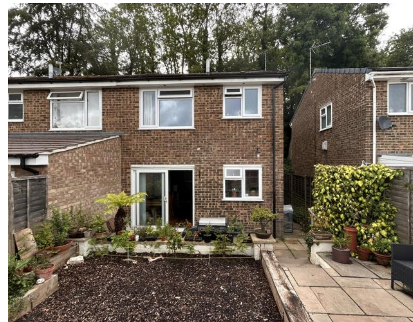
Rear view of No.28
