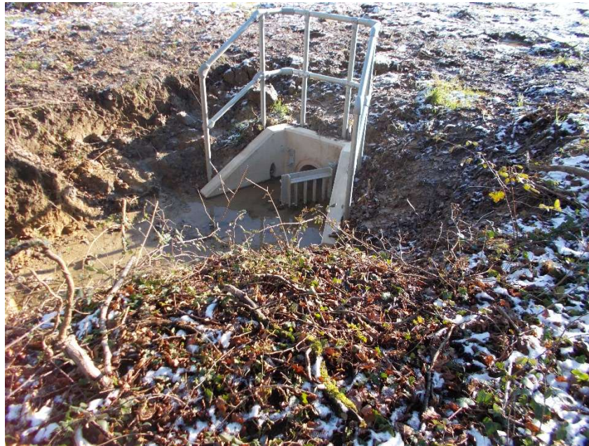
Drainage construction on Taylor Wimpey site (ditch on the eastern site boundary - greater than 5m from the construction on Site A)
