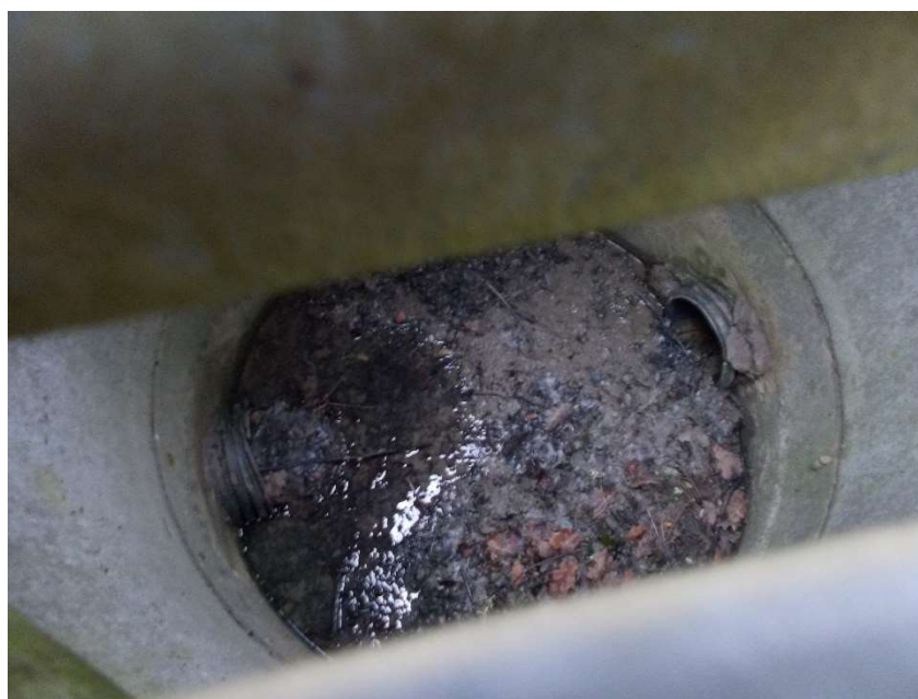
Internal view of the 1 st chamber
