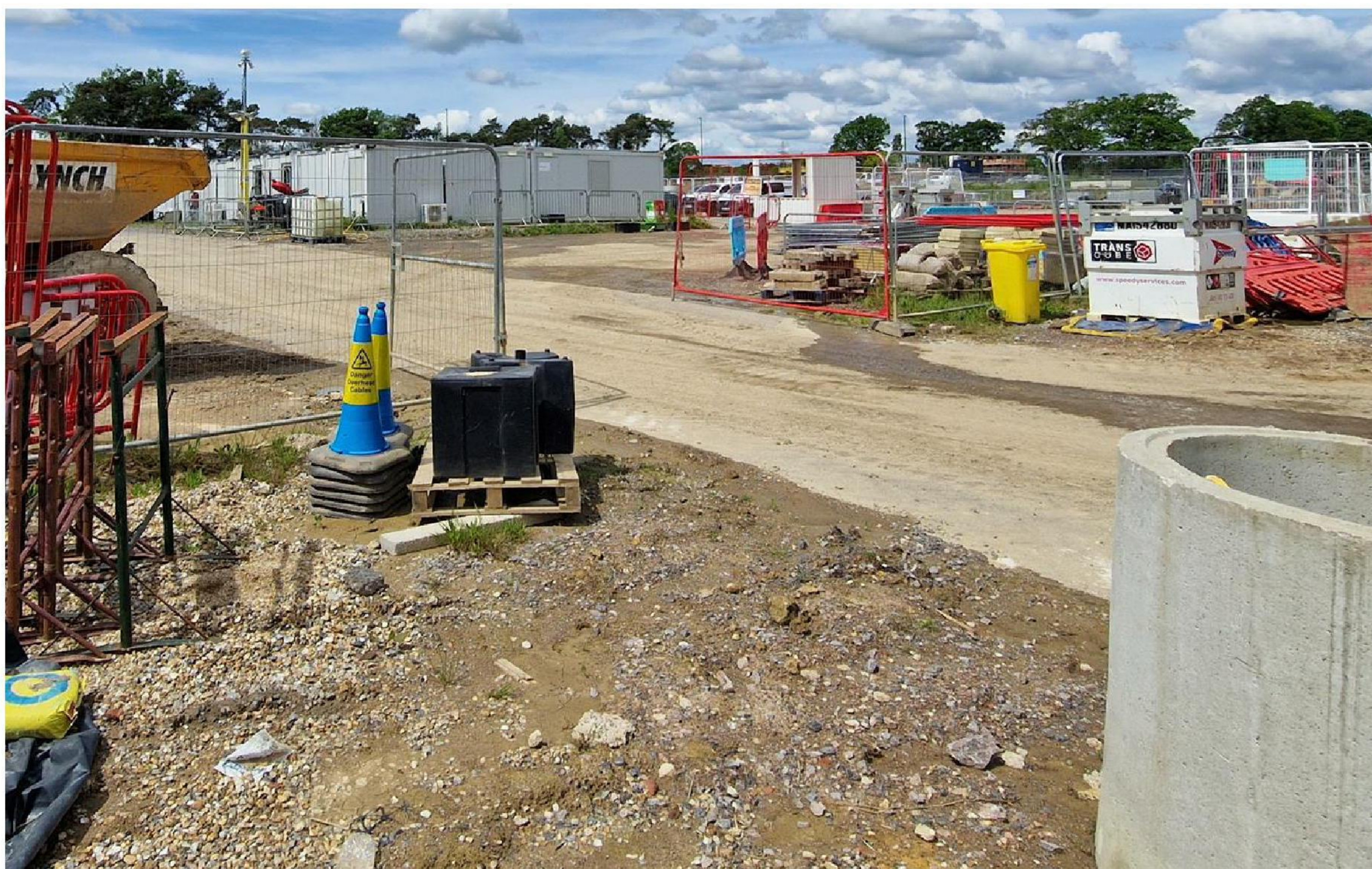
Figure 10: u1c artificial unvegetated unsealed surface (construction compound)
