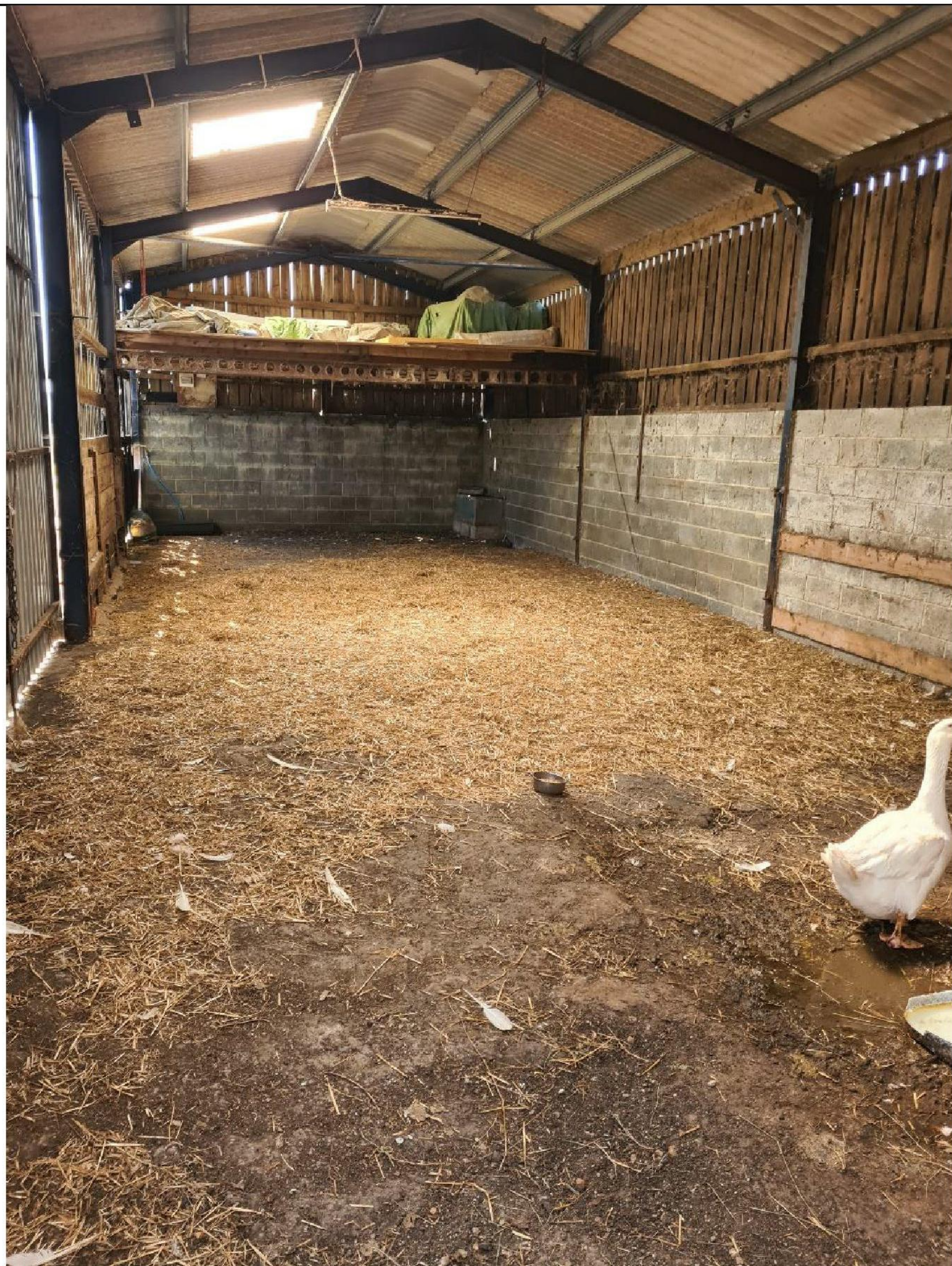
Figure 2. The interior of the southern part of the building.
