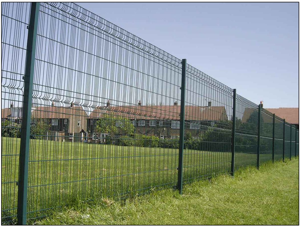
Example of existing Paladin fence fencing 1800mm.
