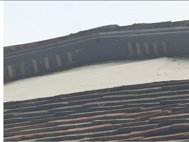
Picture 6: Damaged eaves and lifted hanging tiles on the northern elevation of B2
