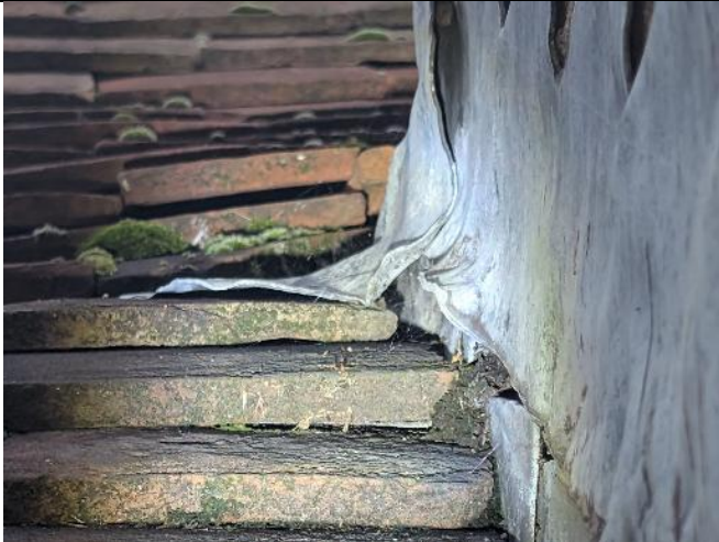
Picture 7: Lifted tiles and lead flashing on B2
