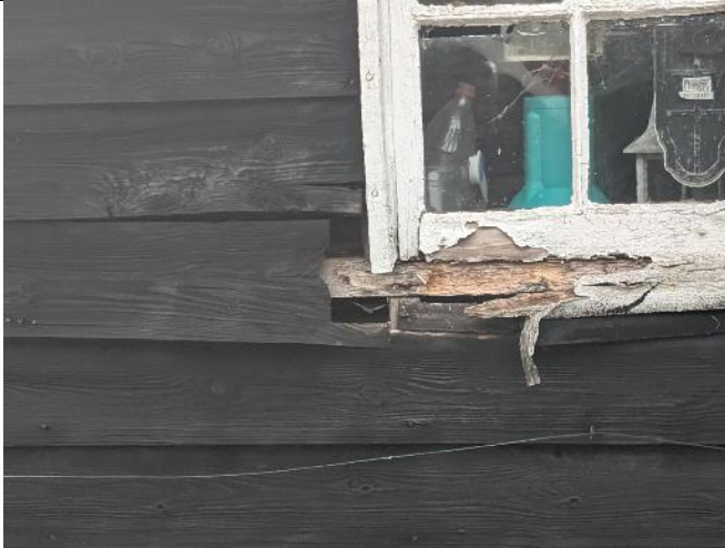
Picture 13: Damage and gaps around window B4
