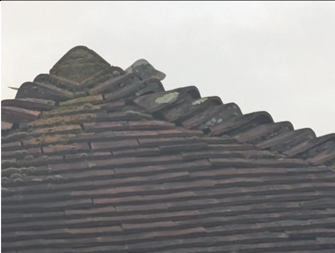
Picture 11: Missing mortar and lifted roof tiles on B3
