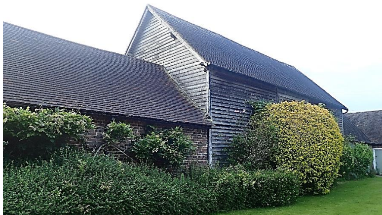
Fig. 2 – The barn, viewed from the south-east
