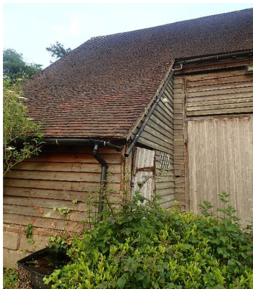
Fig. 4 – the barn, showing NW lean-to
