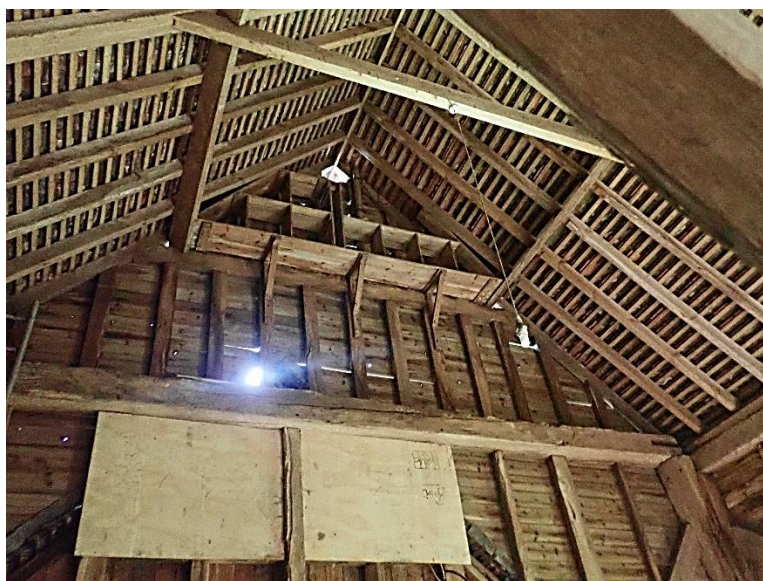
Fig. 6 – View to south end of barn
