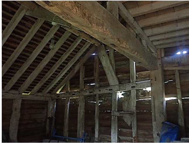
Fig. 7 – View of lean-to room at NW
