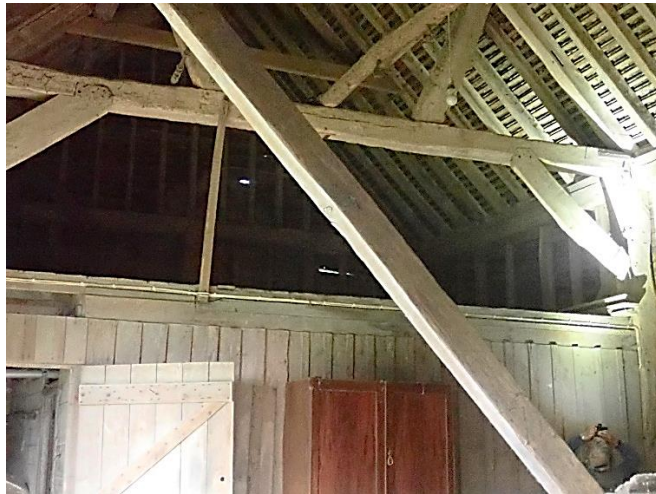
Fig. 8 – View to mezzanine floor at N
