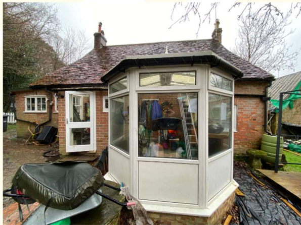
Figure 8: Expressed brickwork of the rear elevation of the original part of the cottage viewed through the modern conservatory
