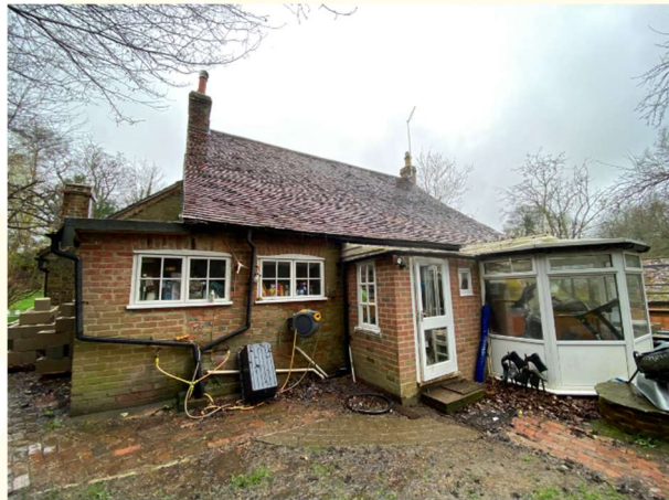
Figure 7: 20 th century kitchen extension, brick porch and conservatory to the rear of Rowfant Mill Cottage
