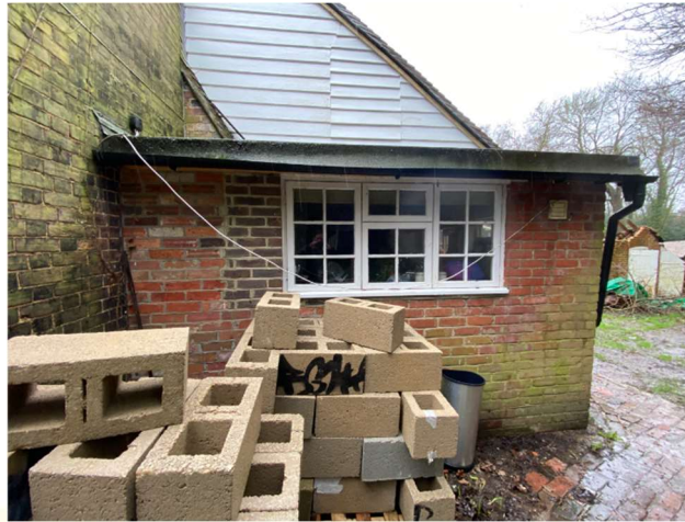
Figure 6: Mid-late 20 th century kitchen extension
