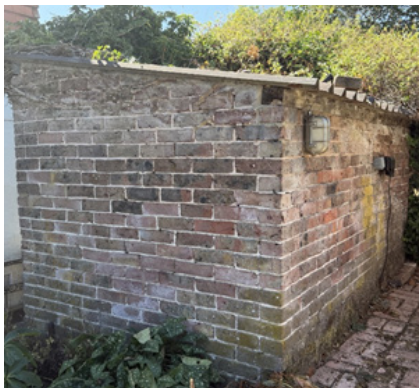
Retaining wall built from reusing existing sandstone blocks and recycled bricks from demolished outhouse
