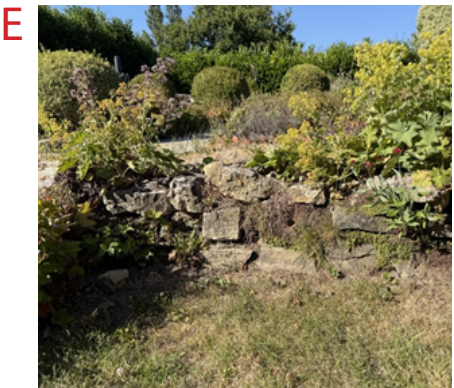
Retaining wall built from reusing existing sandstone blocks and recycled bricks from demolished outhouse
