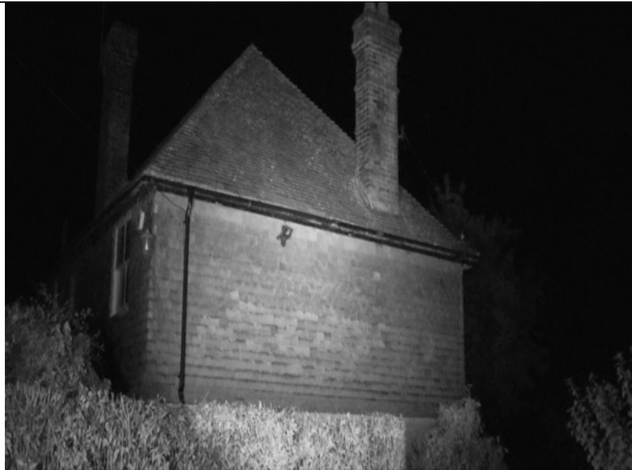
Photograph 2: Northwestern aspect of the building at darkest point of survey (15/09/26)
