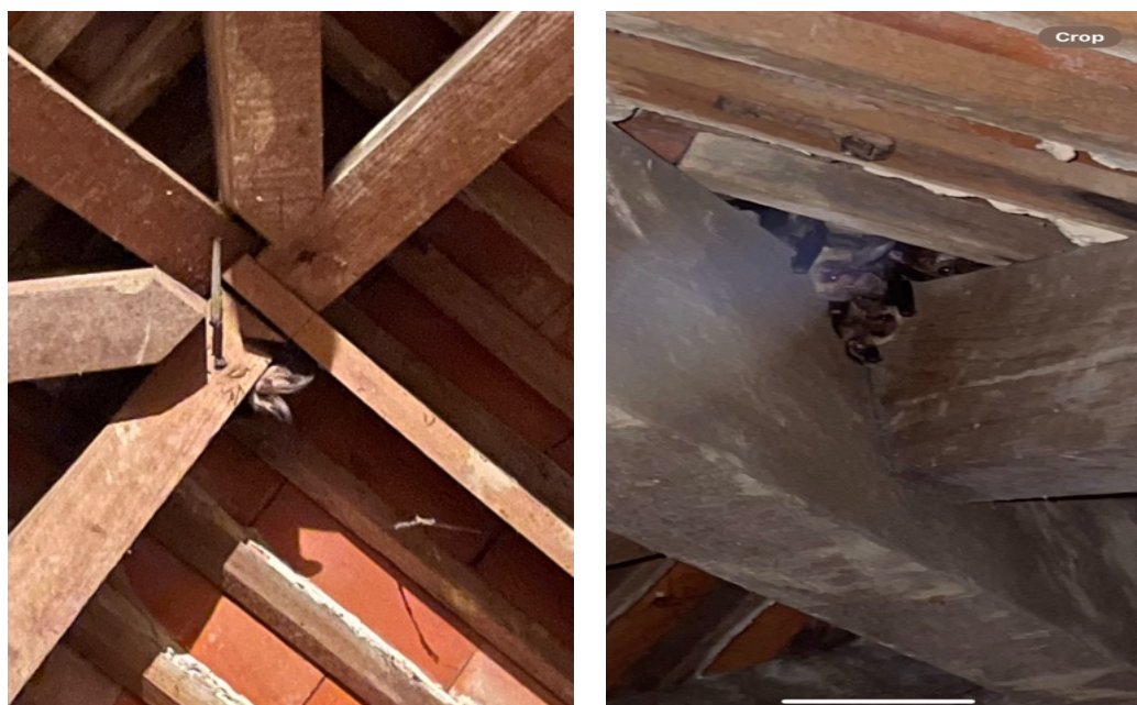
Figure 5: Brown long eared bats recorded in roof void
