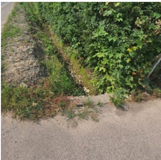
Figure 2a: Ditch (looking north on Cuckfield Road)
