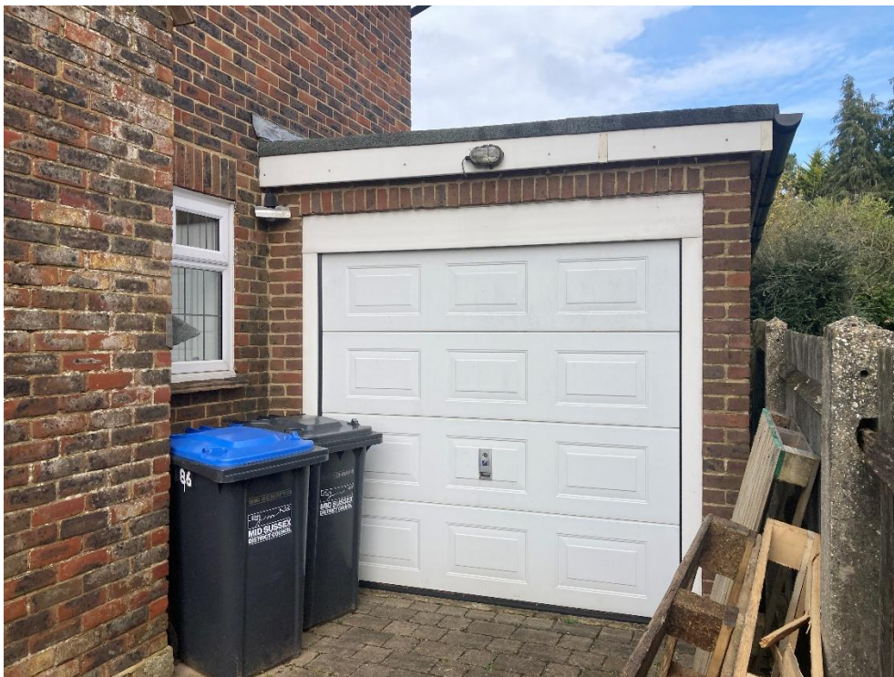
Image 05 – Existing front elevation of the non-original garage proposed to be demolished.
