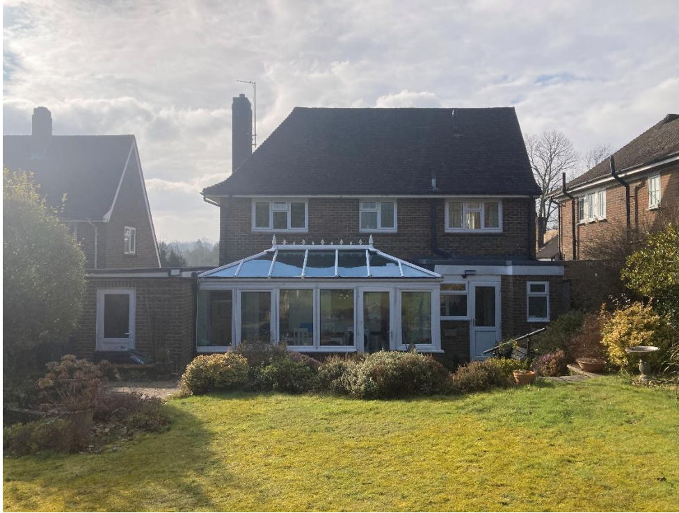
Image 02 – Existing rear elevation of number 86 Harlands Road.
