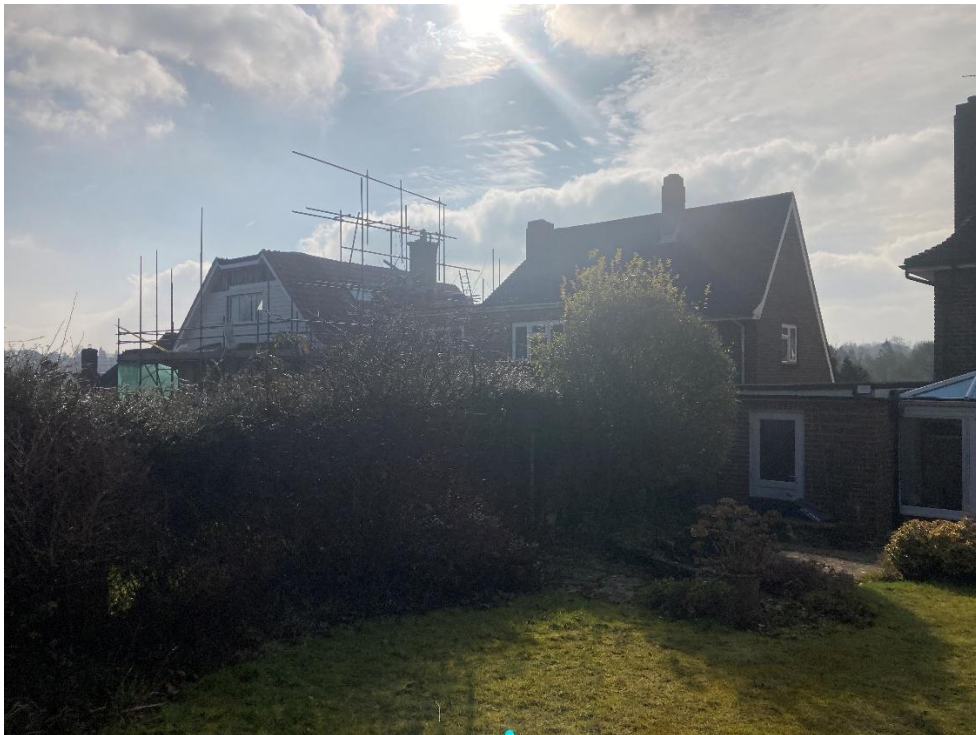
Image 03 – Existing rear elevation of numbers 82 and 84 Harlands Road, viewed from number 86's rear garden.
