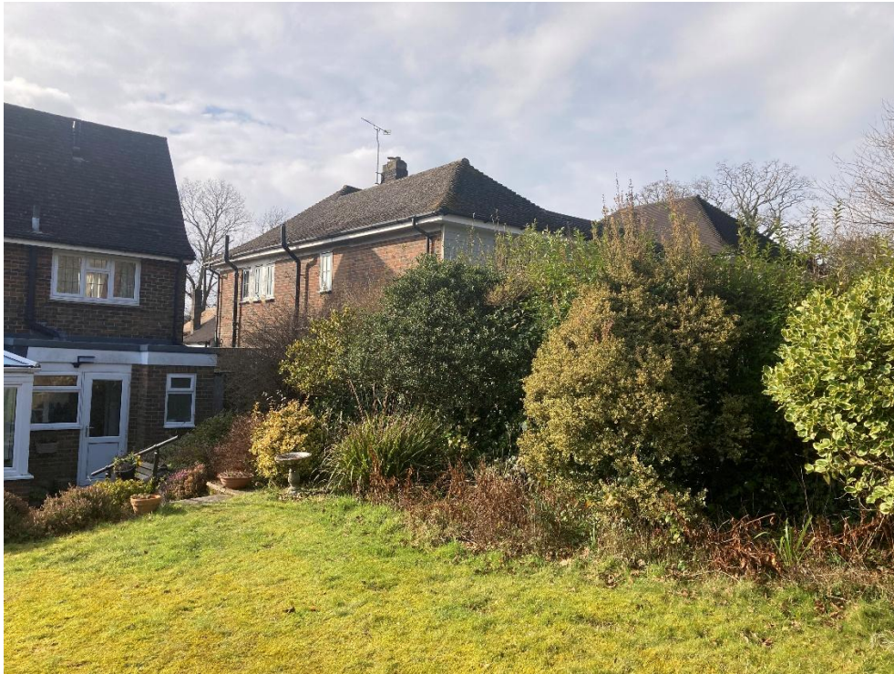
Image 04 – Existing rear elevation of number 88 Harlands Road, viewed from number 86's rear garden.
