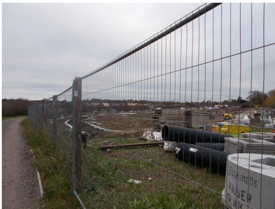
Taylor Wimpey construction site showing path/location of foul drainage
