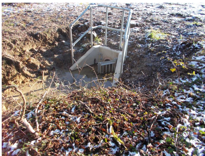
Drainage construction on Taylor Wimpey site (ditch on the eastern site boundary - greater than 5m from the construction on Site A)
