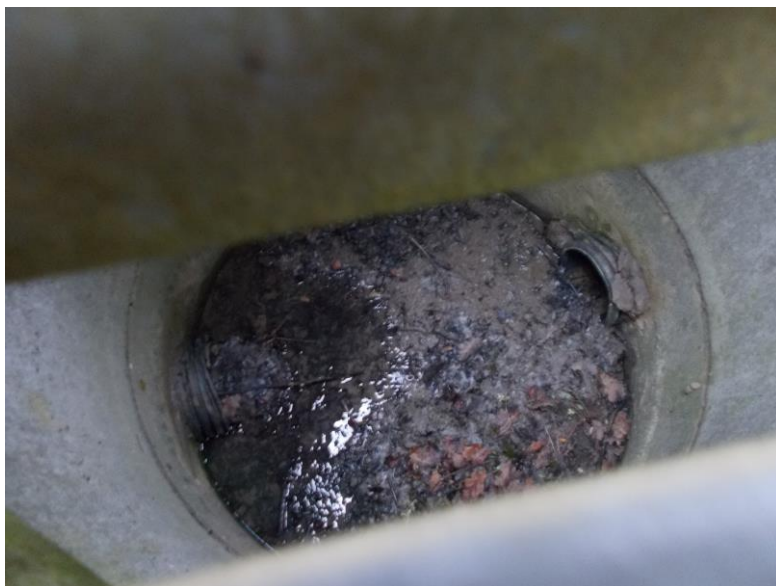
Internal view of the 1 st chamber
