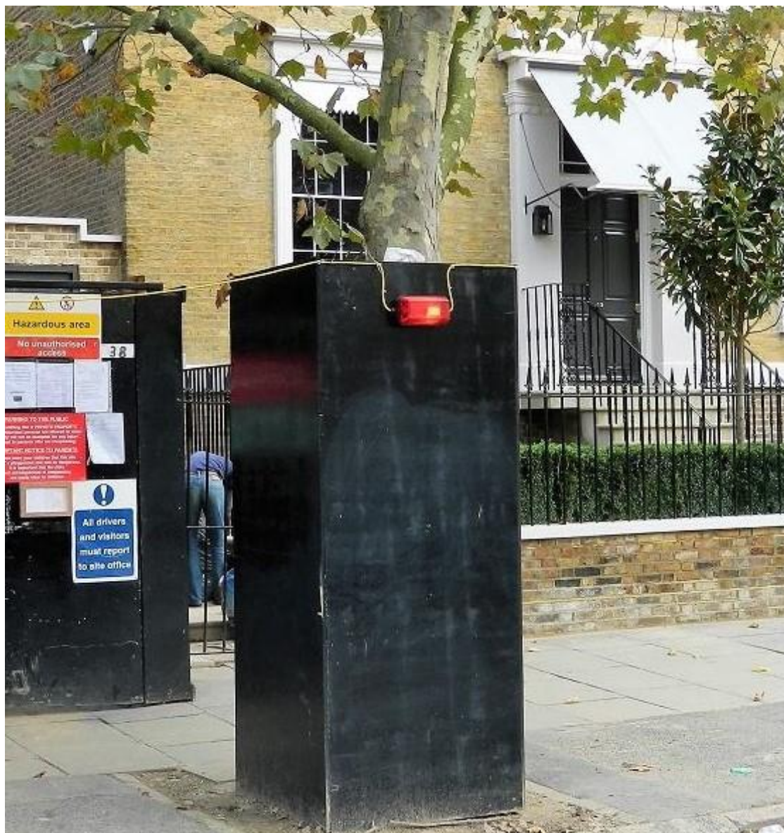
Figure 6 Example of Box Hoarding
