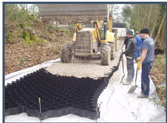
Figure 12 Examples of Cellweb filling with angular stone
