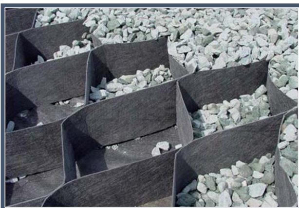
Figure 12 Examples of Cellweb filling with angular stone
