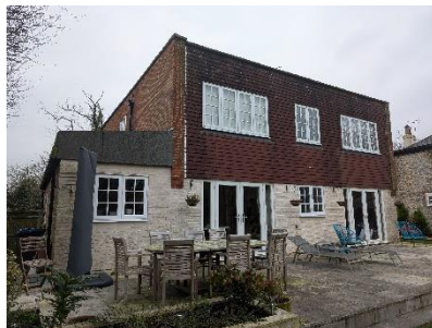
Rear of existing dwelling
