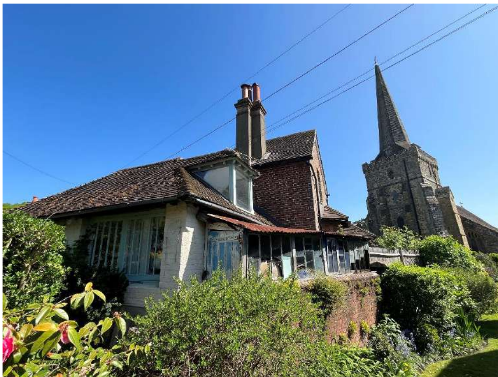
Photo Above: The rear elevation of Mason Cottage which consists of a lean-to outhouse/shed to the boundary wall and a dormer window which is blocked up. Mason Cottage's orientation is facing southwest towards Church Platt.
