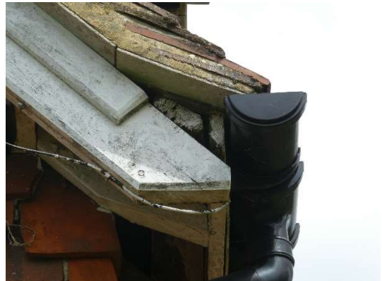
Photograph 4: Missing mortar at south facing tile verge.
