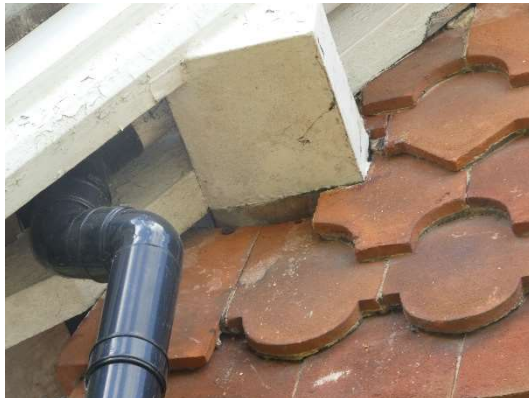
Photograph 3: Gap at the eaves associated with the north elevation.
