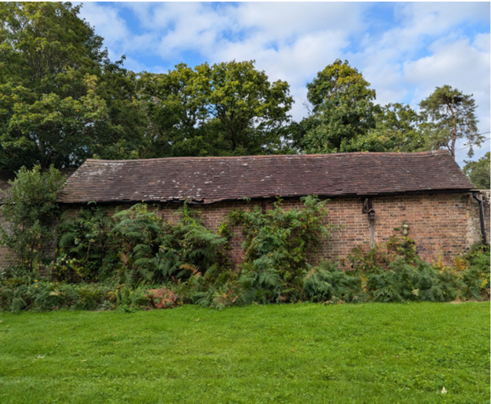
South side of Shed
