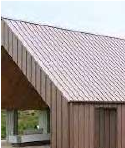
7. Zinc standing seam roof
