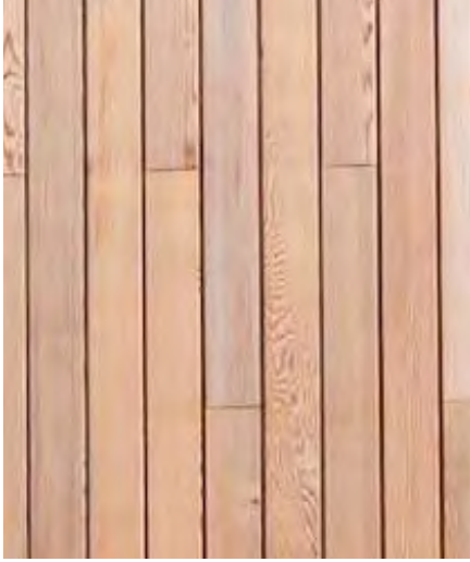
4. Vertical timber cladding
