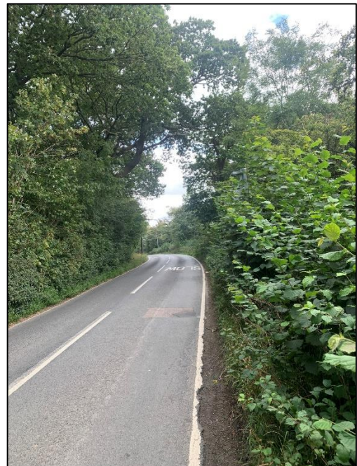
Photograph 2: Hanlye Lane westbound
