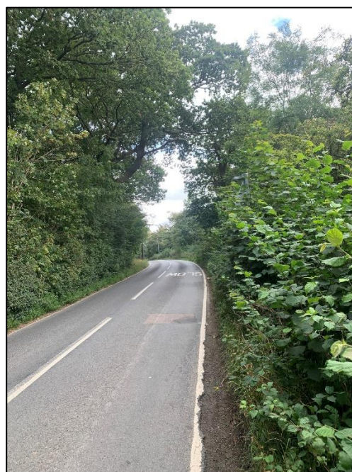
Photograph 2: Hanlye Lane westbound
