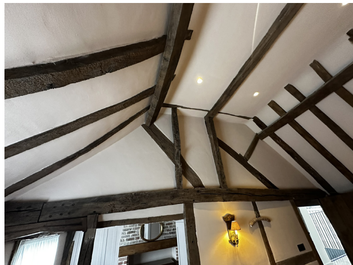
First Floor - historic timber frame roof
