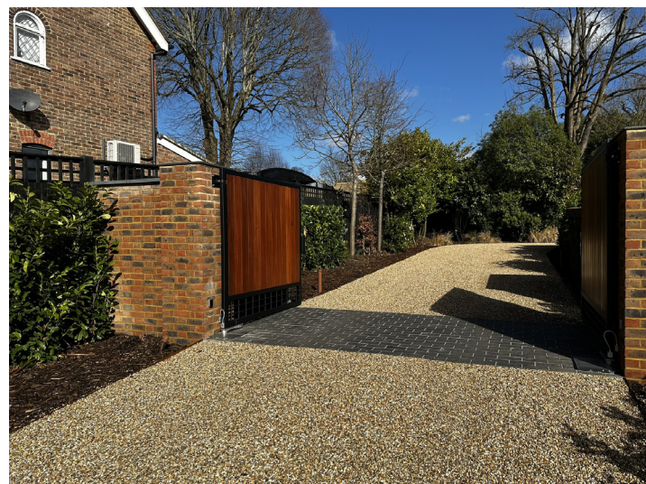
Gravel driveway and new gates
