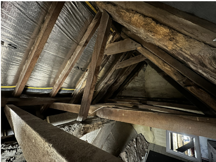
Attic - historic timber frame roof
