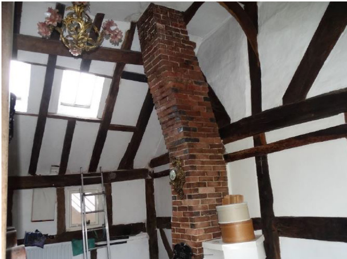
First floor bedroom, chimney stack
