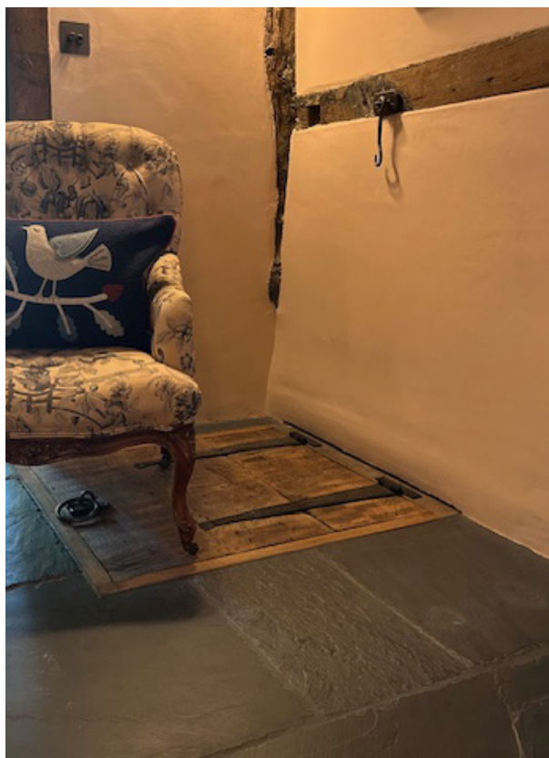
Ground Floor -access hatch to basement
