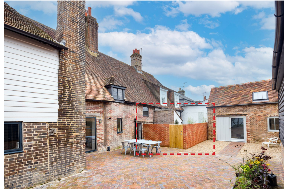
As-built rear brickwork wall
