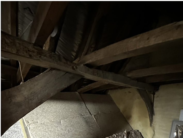
Attic - historic timber frame roof
