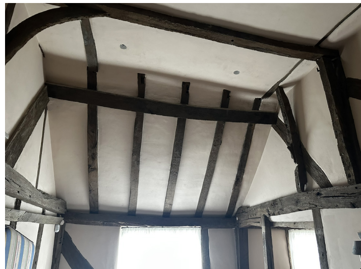
First Floor - historic timber frame roof
