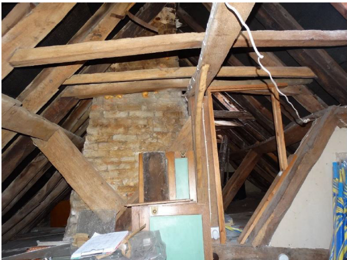
Attic, chimney stack in the background
