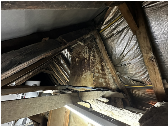
Attic - historic timber frame roof
