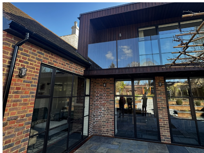
Rear elevation & re-constructed bake house
