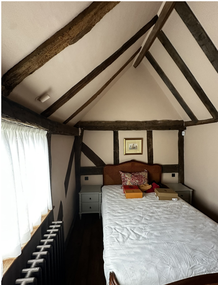
First Floor - historic timber frame roof
