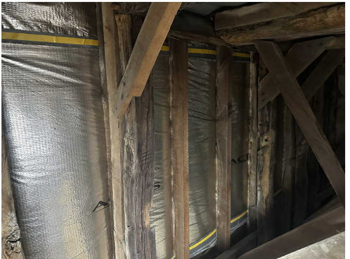
Attic - historic timber frame roof, new insulation
