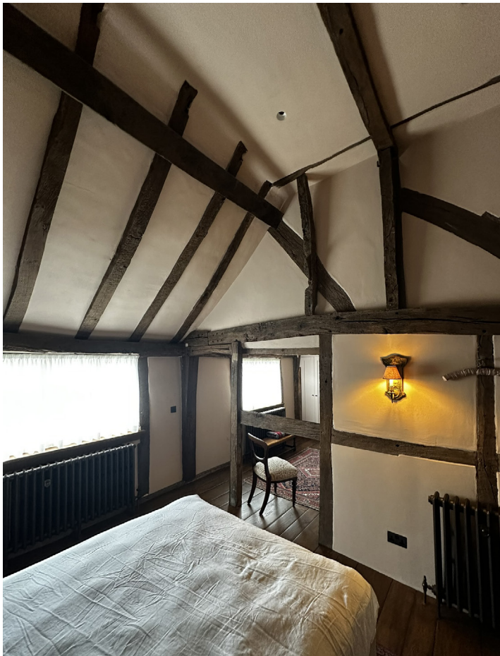
First Floor - historic timber frame roof
