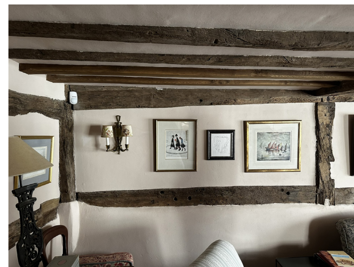
Historic timber frame wall, living room
