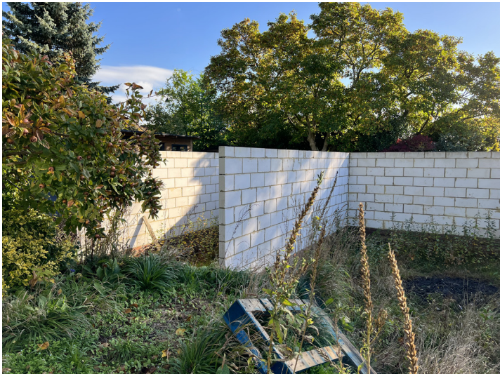
Garage walls constructed
