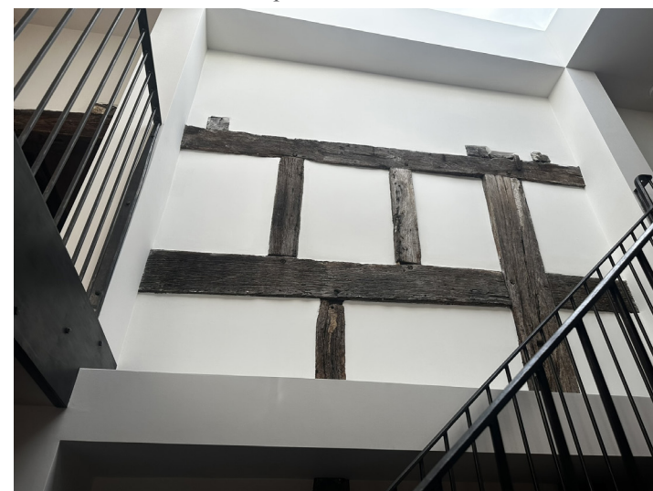
Historic timber frame wall in stairwell
