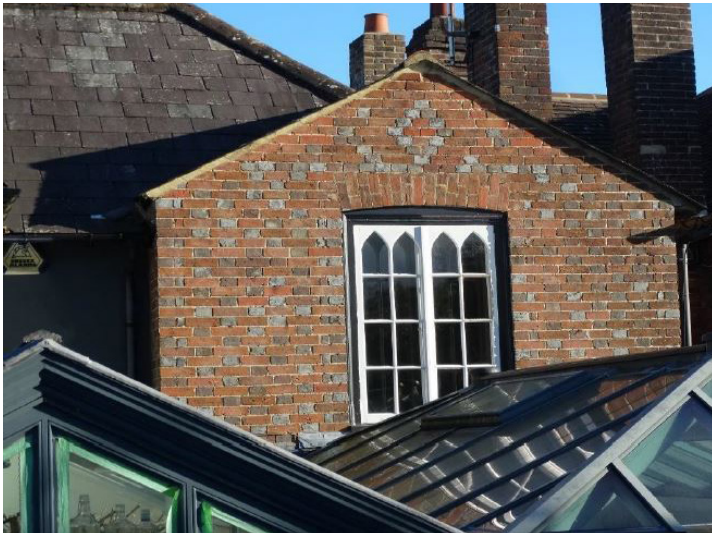
Historic rear extension with gothic window
