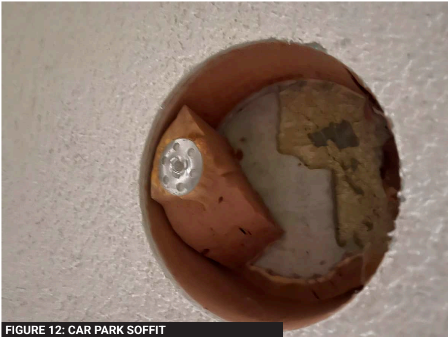
FIGURE 12: CAR PARK SOFFIT
