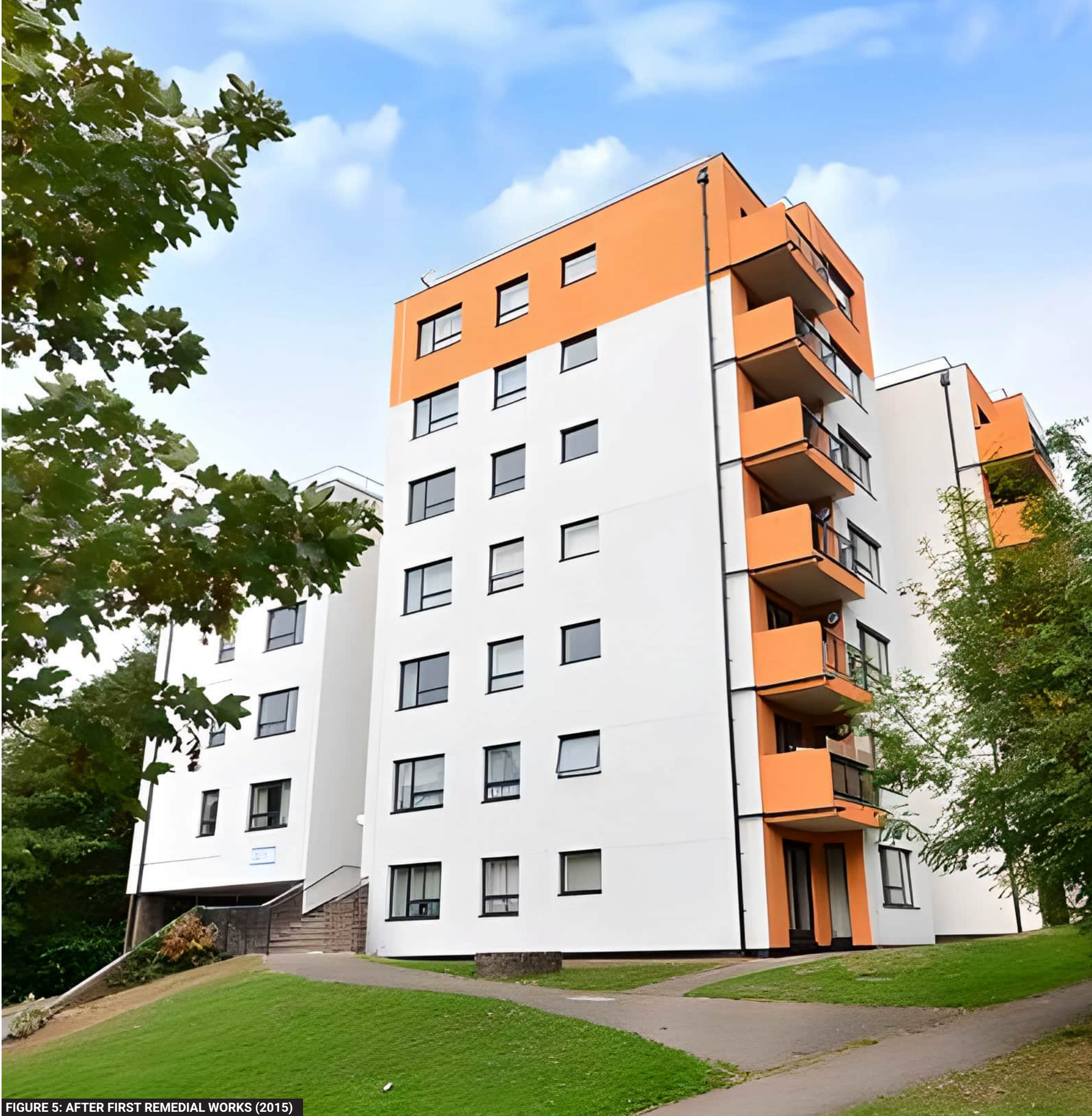
FIGURE 5: AFTER FIRST REMEDIAL WORKS (2015)
