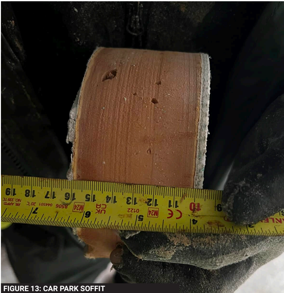
FIGURE 13: CAR PARK SOFFIT
