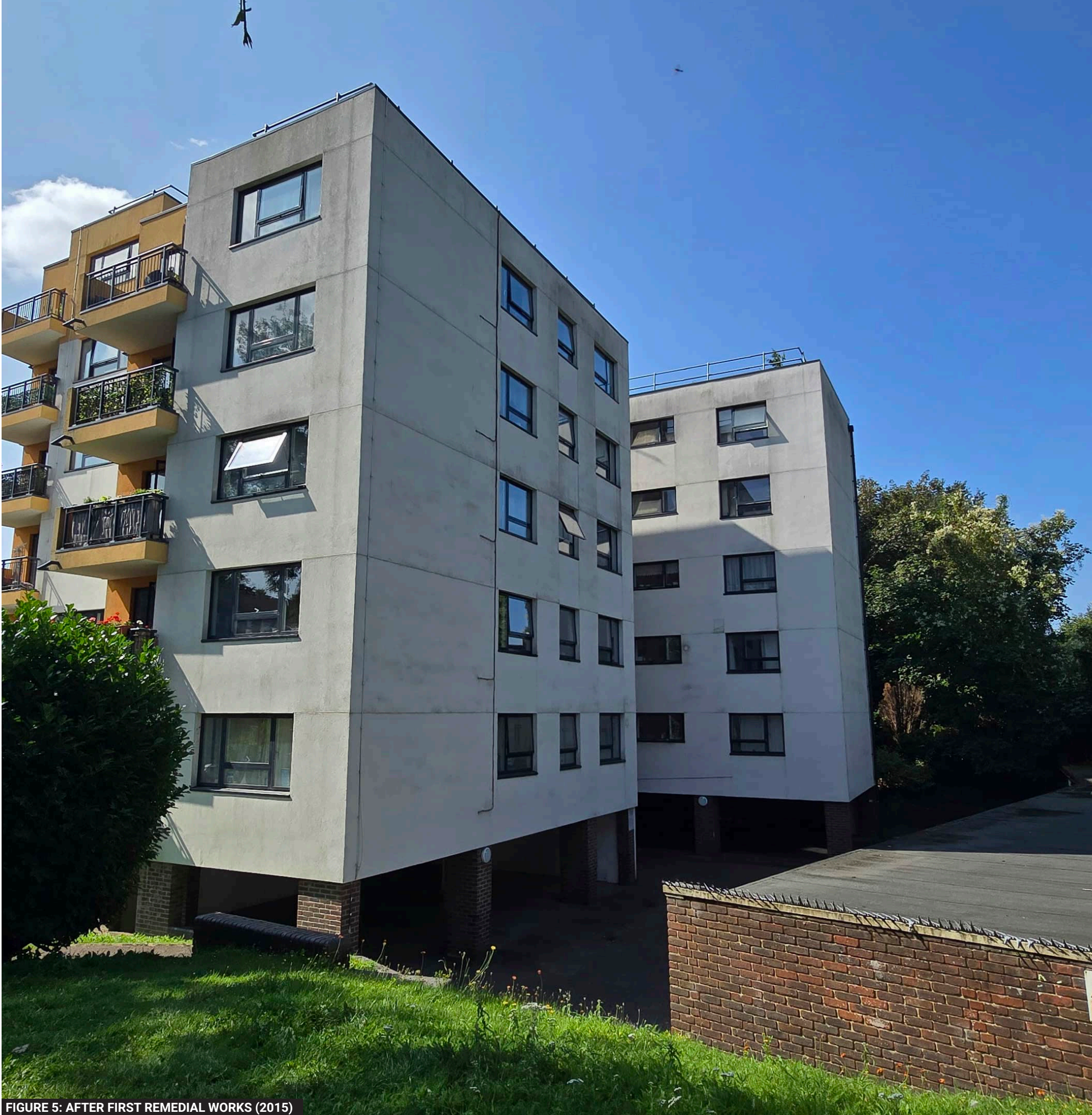
FIGURE 5: AFTER FIRST REMEDIAL WORKS (2015)
