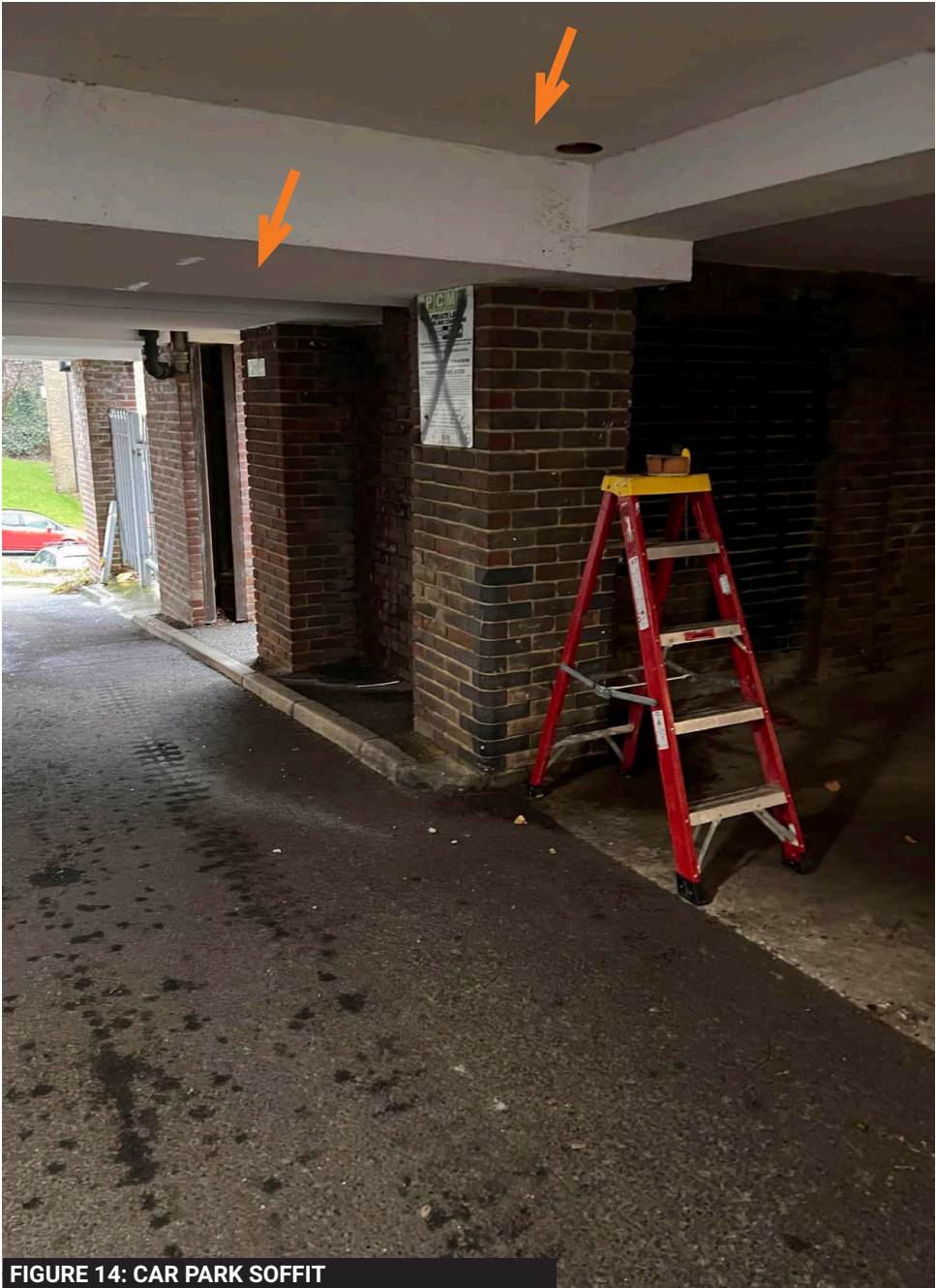
FIGURE 14: CAR PARK SOFFIT
