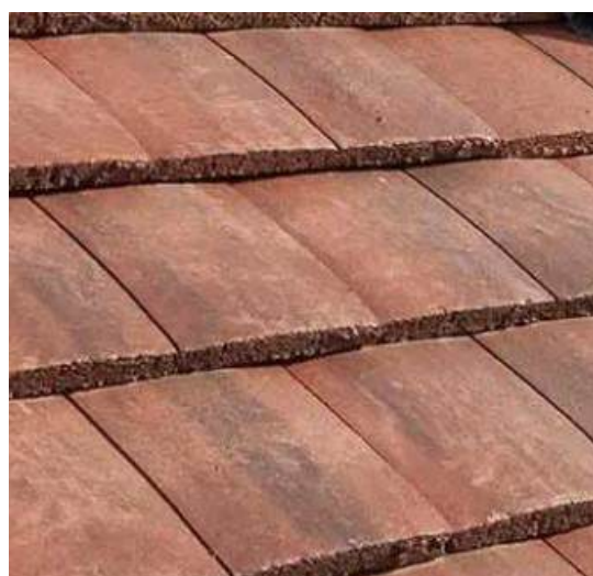
4. ROOF - CONCRETE TILE (SOUTH ELEVATION ONLY)
