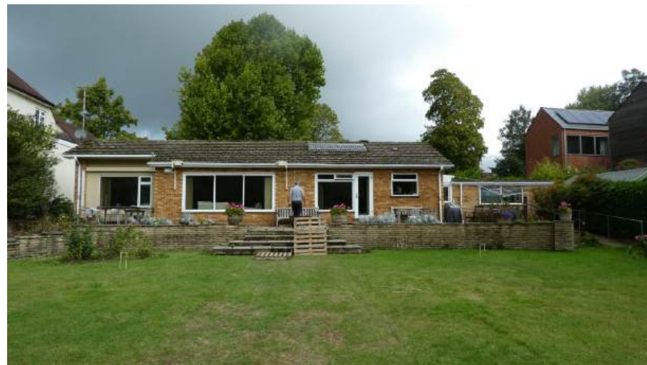
4. View of rear
