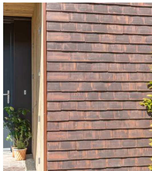
2. WALLS (UPPER) - CLAY TILE HANGING
