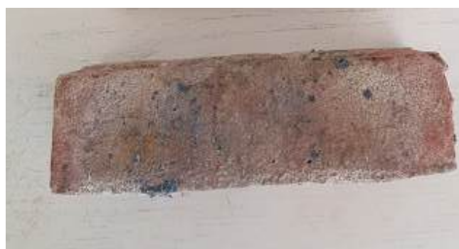
1. WALLS (LOWER) - LOCAL STOCK BRICK
