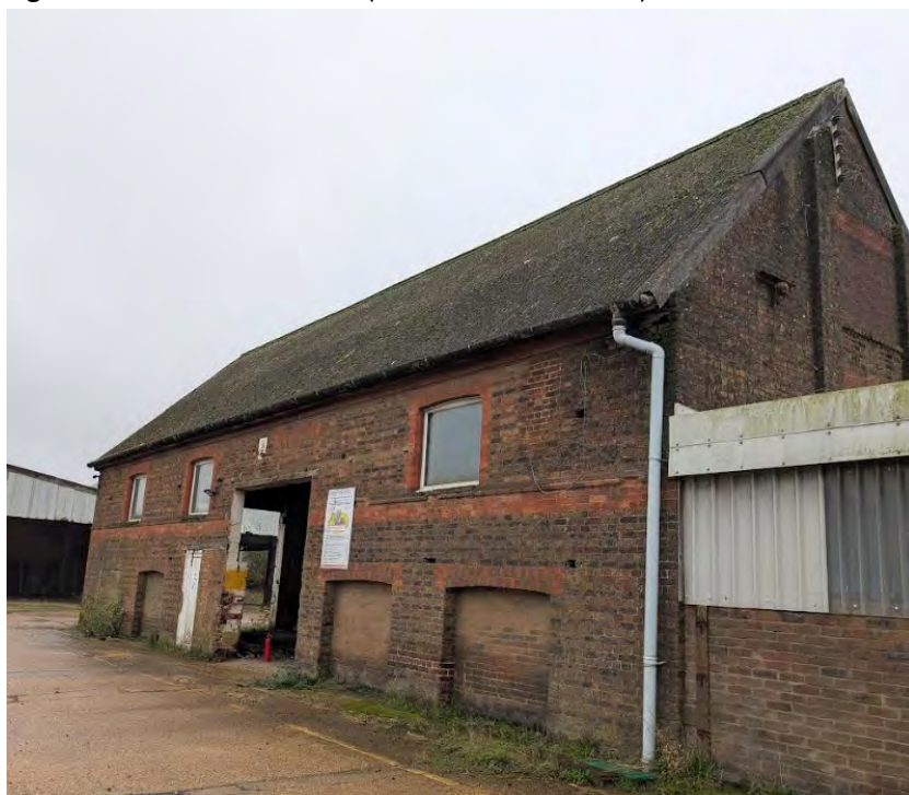
Figure 10. View of B4a on site (taken November 2024).
