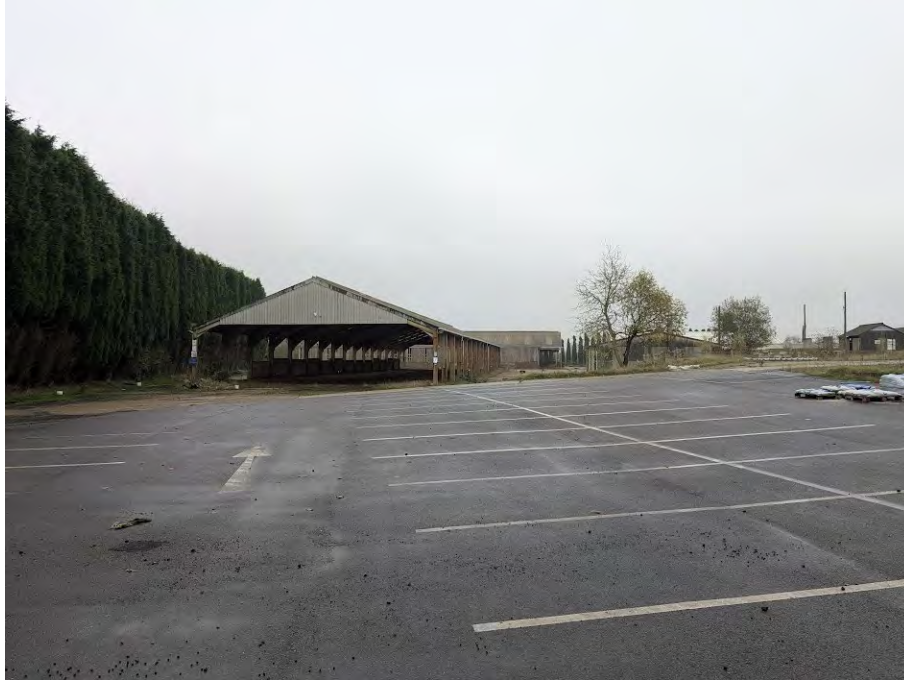
Figure 3. Example of the developed land and buildings on site (taken November 2024).
