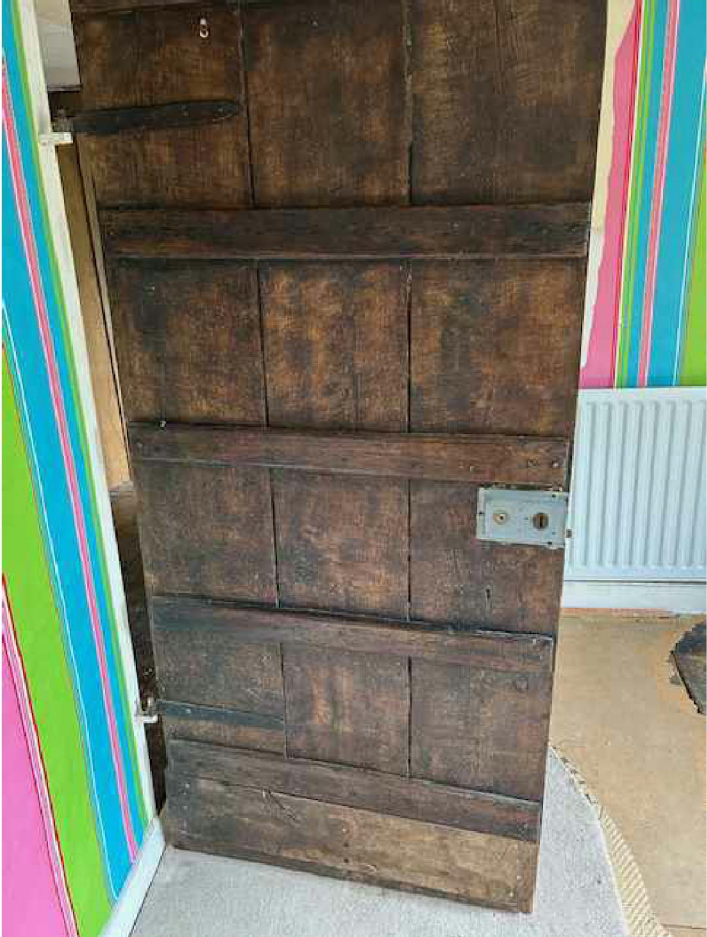
Existing timber door to be re-instated and fixed shut
