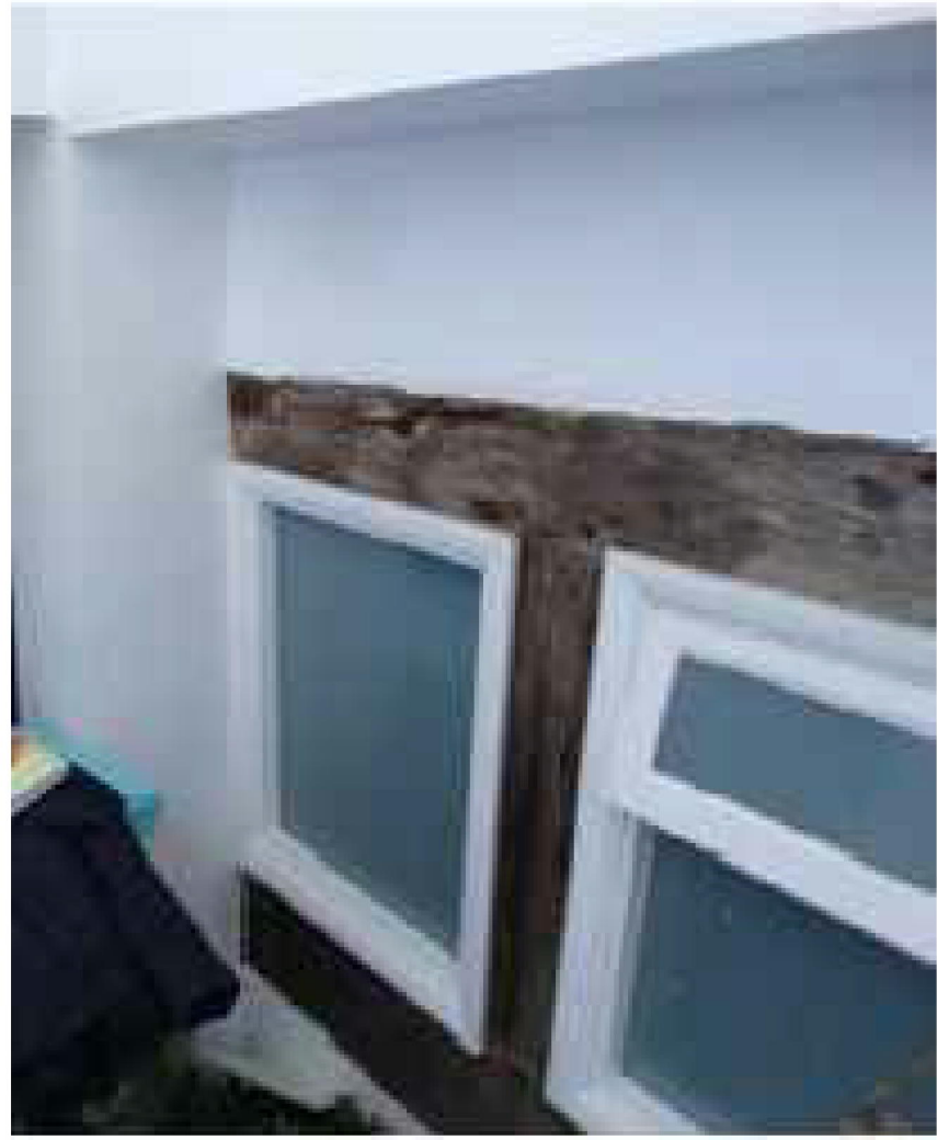
Before: uPVC casement windows before removal
