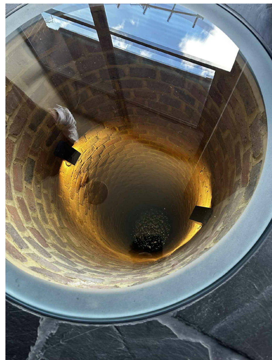
Recent photograph of the well shaft
