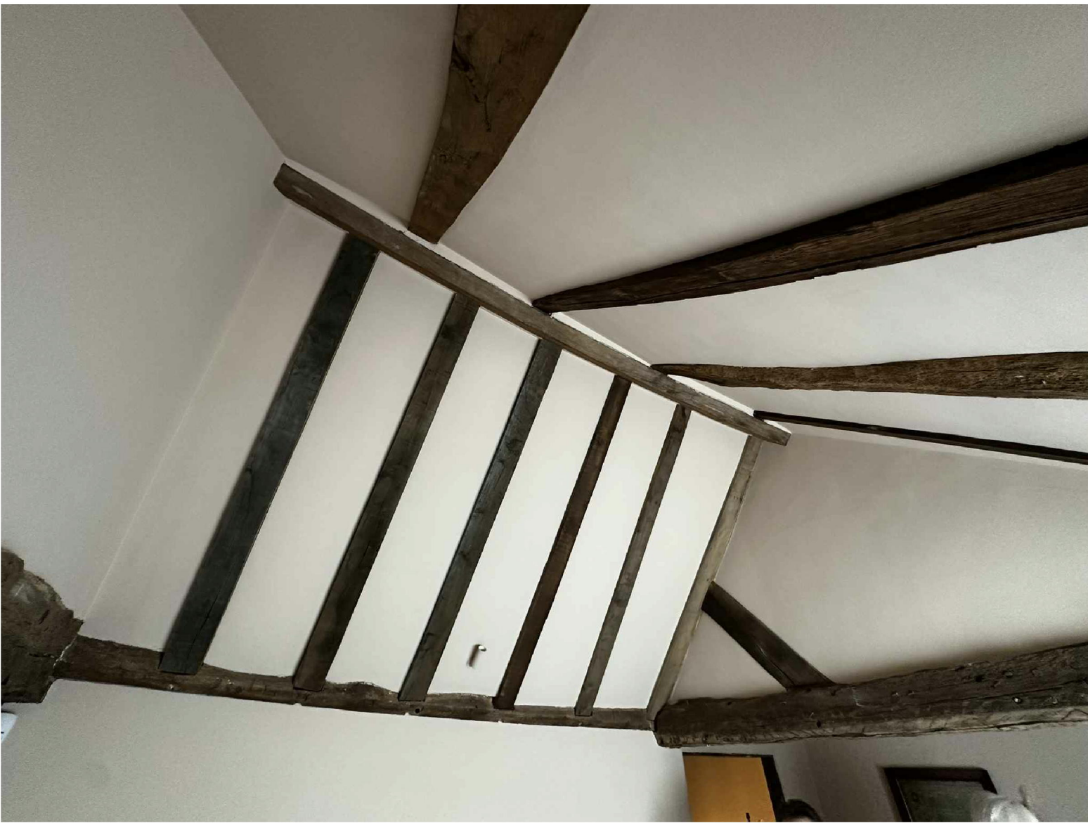
Vaulted ceiling, first floor SE bedroom
