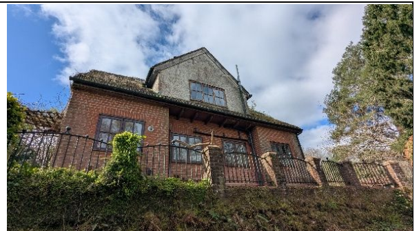
Photo 2: The southeast facing elevation of the property.
