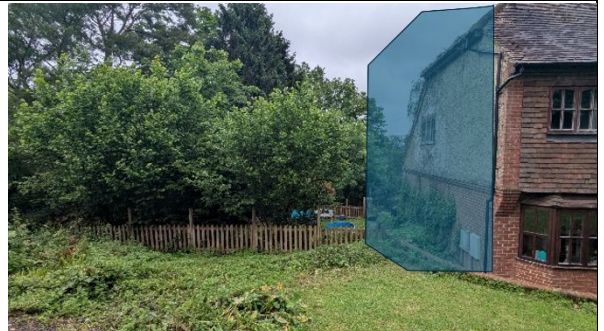
Photo 6: The west elevation, the approximate location of the new extension is indicated (blue shading).
