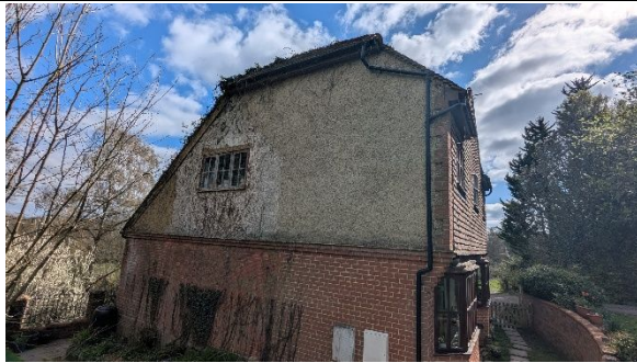
Photo 5: The northeast facing elevation of the property where the extension will be attached.
