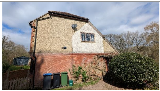
Photo 4: The southwest facing elevation of the property.
