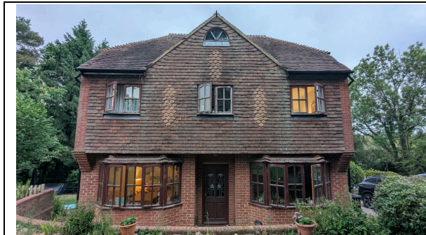
Photo 1: The northwest facing (front) elevation of the property.
