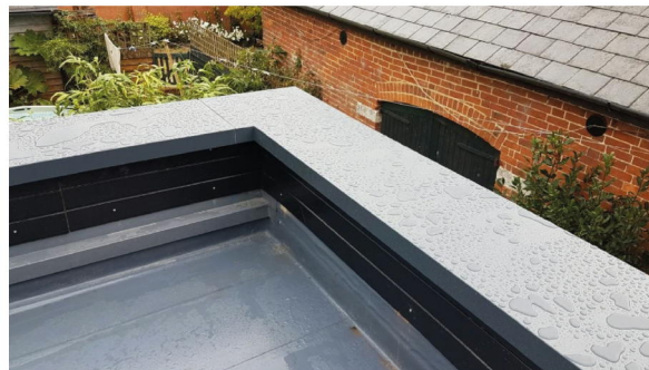
Fig. 2. GRP roof finish with aluminium coping.
