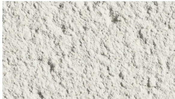
Fig. 4. Through colour monocouche render.
