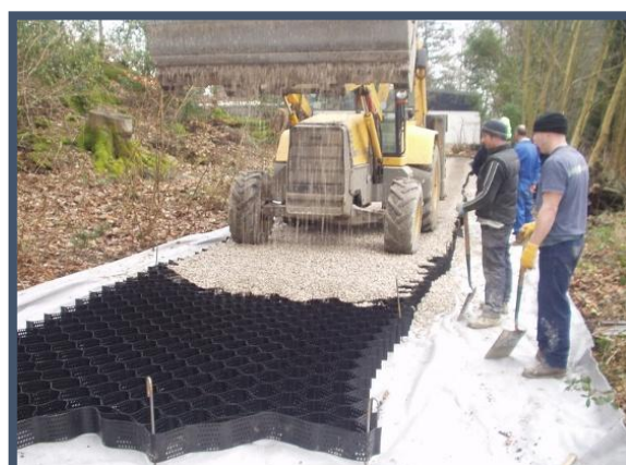
Figure 13 Examples of Cellweb filling with angular stone
