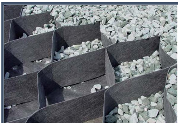
Figure 13 Examples of Cellweb filling with angular stone
