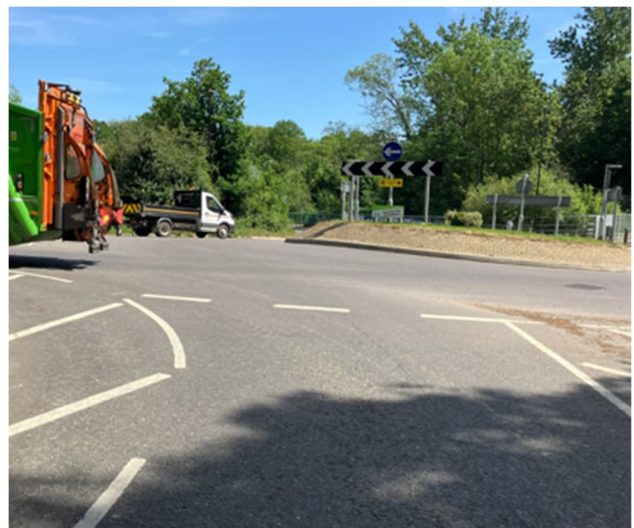
IMAGE: Photo showing restricted forward visibility to Fairbridge Way from Cuckfield Road due to central roundabout island.
