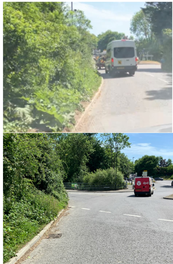
IMAGE: Photos showing dense vegetation on eastern side of Isaac's Lane, restricting forward visibility to Fairbridge Way.
