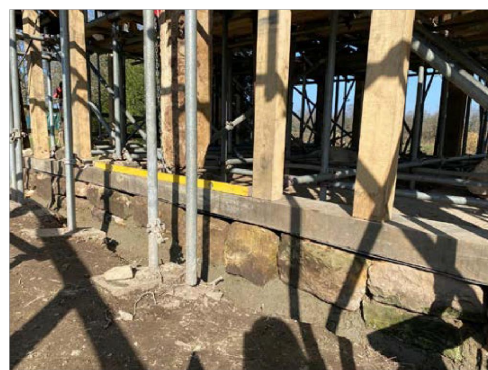
New oak wall members morticed into new sole plate. (Original members too rotten to replace), on reinstated stone plinth.
