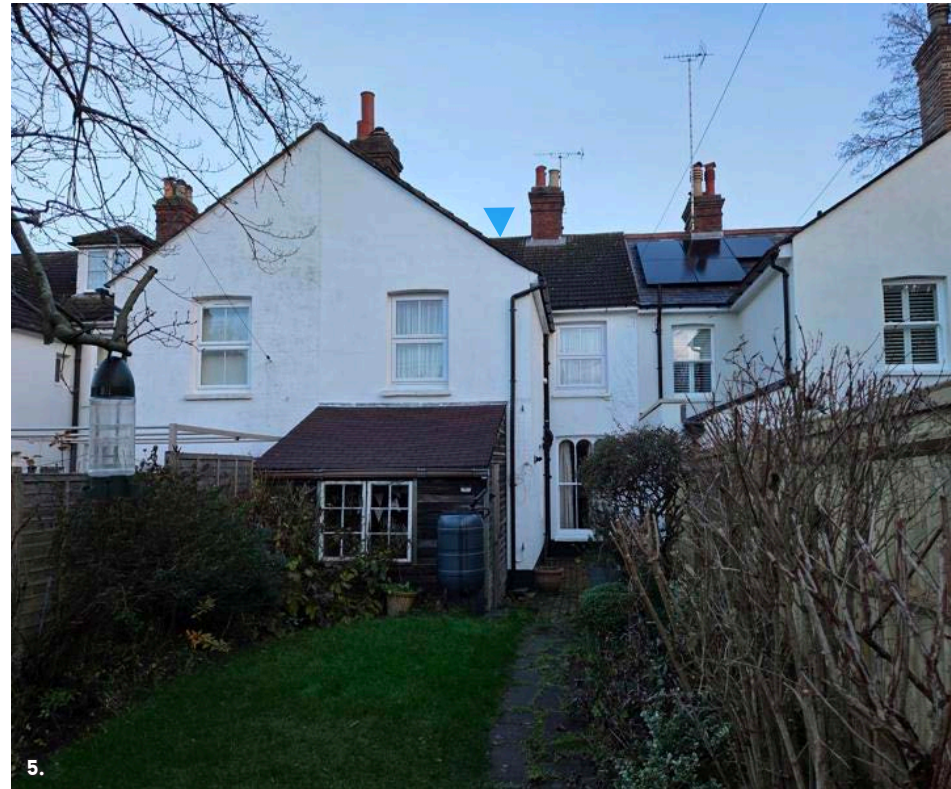
Fig. 15: Rear Garden - Existing white rendered walls and non-original standard double-glazed UPVC windows.
