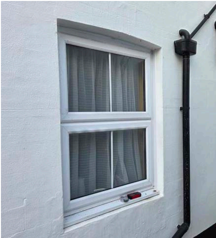
Fig. 37: Photograph of existing UPVC casement window to be replaced.
