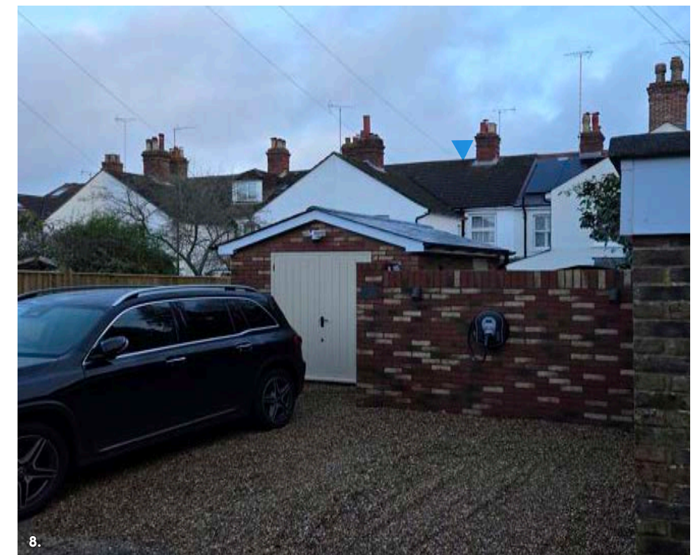
Fig. 18: Rear Access - Example of neighbouring parking / modern garage arrangements. Showing garage at No 142.
