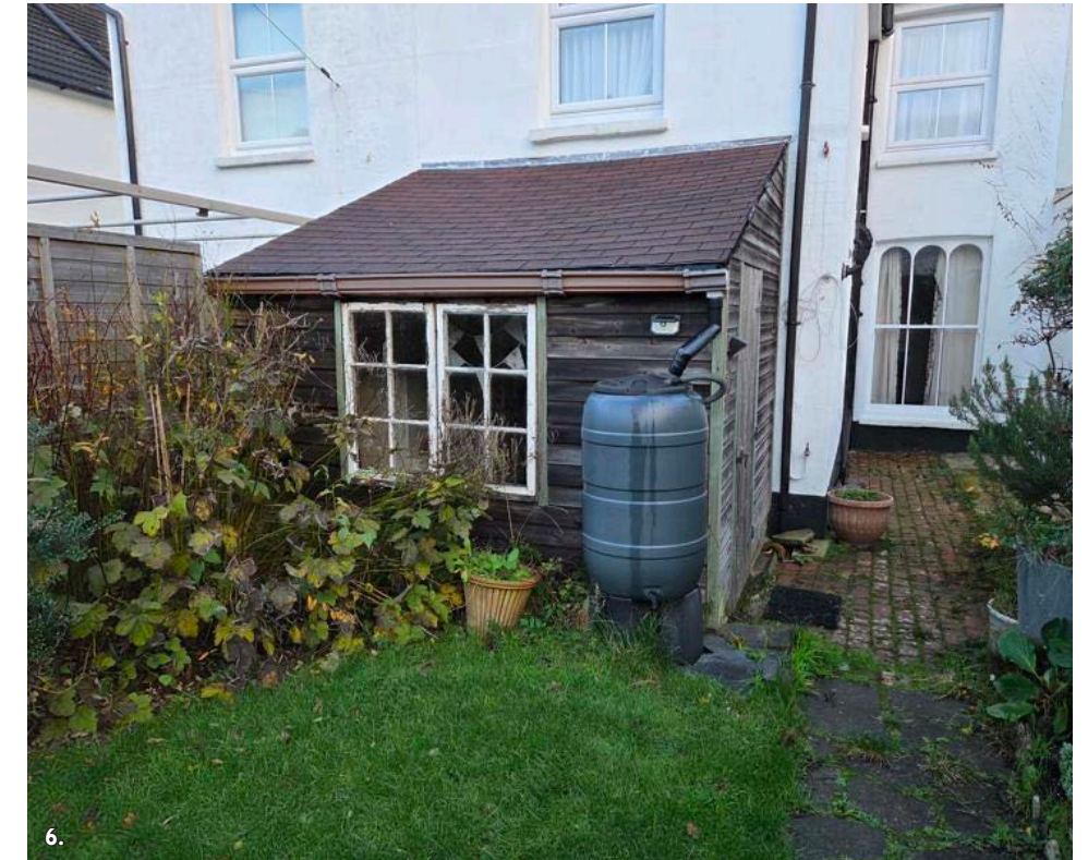
Fig. 16: Rear Garden - Existing lean-to extension proposed for demolition, and hardlandscaped patio area outside of dining room window.
