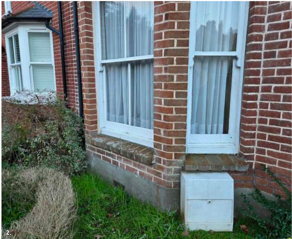
Fig. 11: Front Garden - Existing landscaping & bay window.
