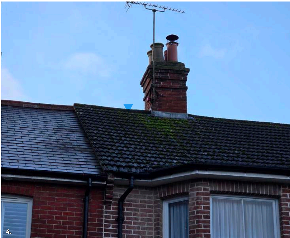
Fig. 12: Front Facade - Existing concrete roof tiles to property and junction with roof slates on neighbours.
