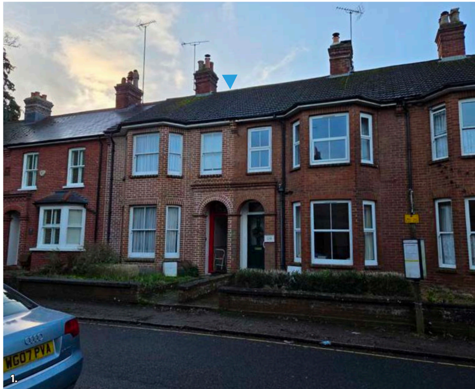
Fig. 10: Front Facade - Main entrance door from High Street
