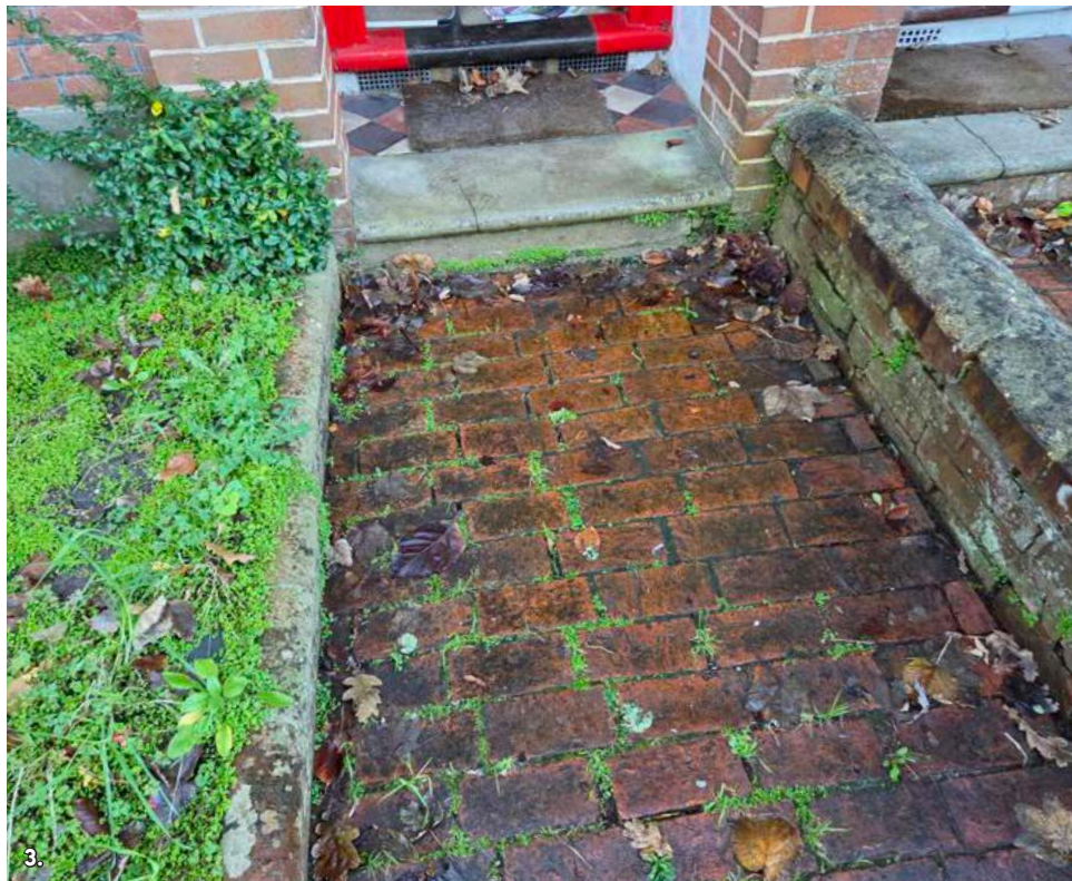
Fig. 13: Front Garden - Existing hard landscaped approach to entrance door.
