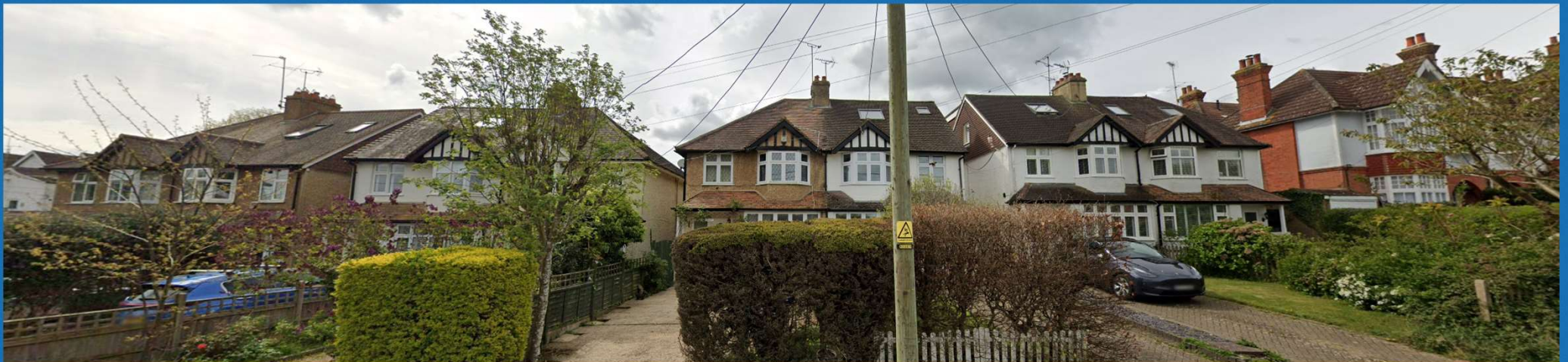
Google Streetview showing No. 36, 38, 40, 46 & 48 hip to gable conversions
