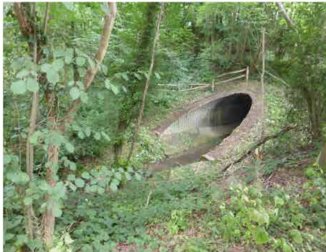
14. View west along lane
