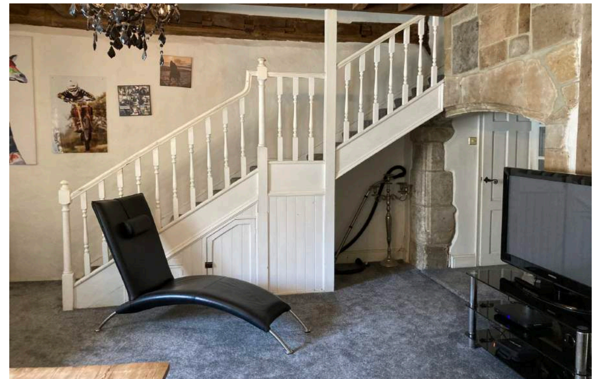
Staircase to be replaced.
