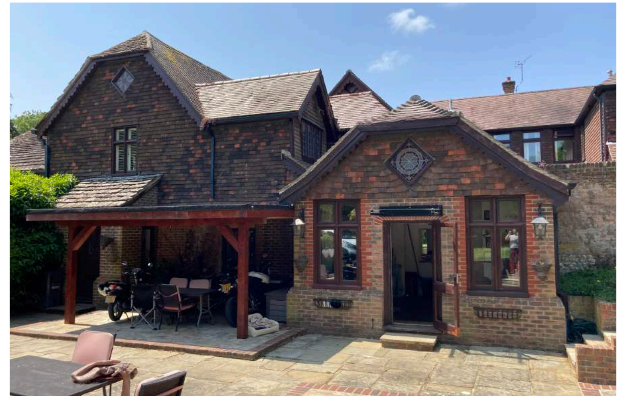
Front (east) elevation of Lyttle Pakyns.
