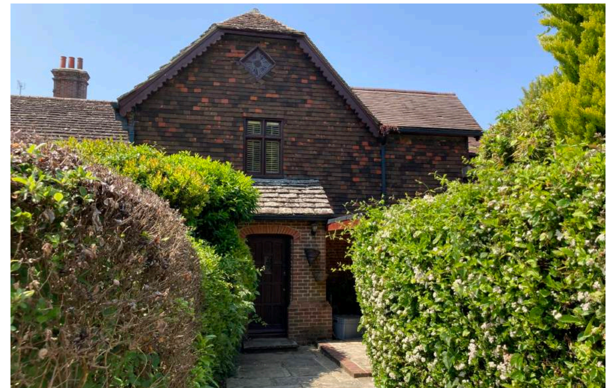
Location of the proposed extension seen from driveway.
