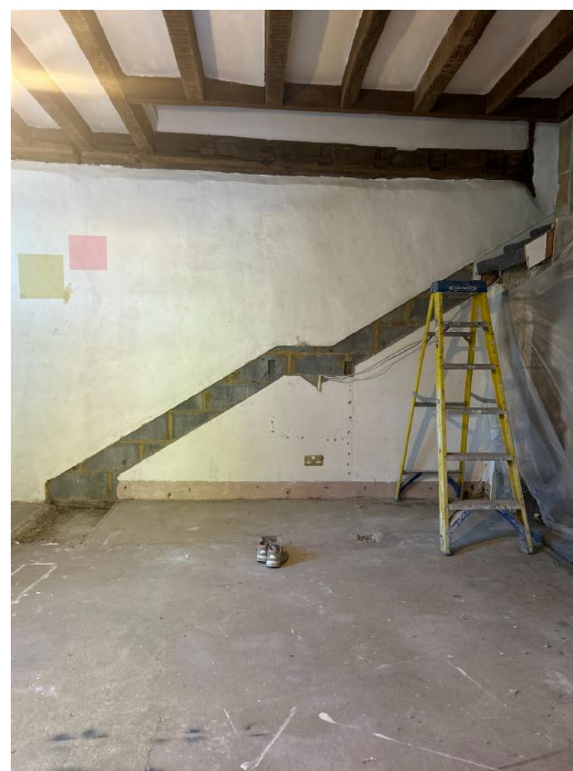
Living Room Interior: photographs show the modern blockwork wall and cracked rough concrete floor prior to the commencement of repairs/works were carried out.
