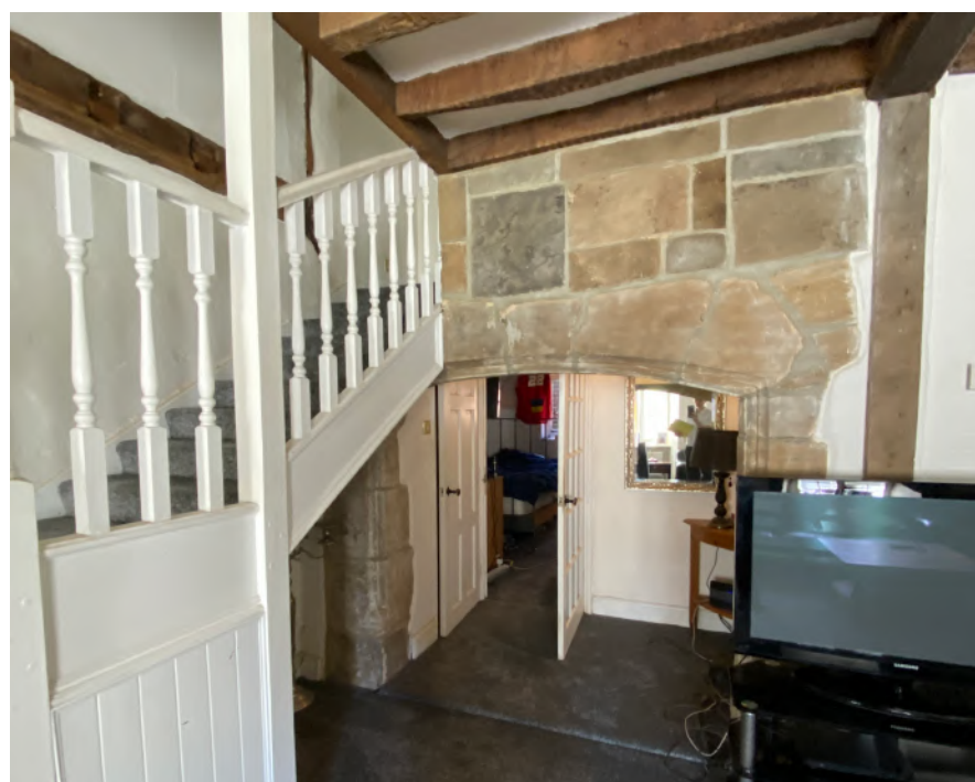
Photograph of fire place prior to commencement of works.
