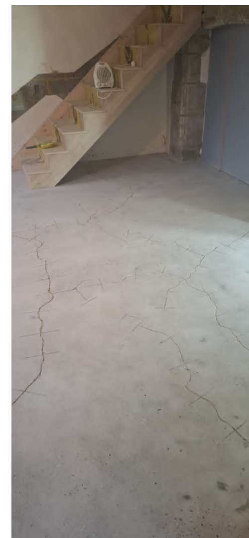
Living Room Interior: photographs show the modern blockwork wall and cracked rough concrete floor prior to the commencement of repairs/works were carried out.
