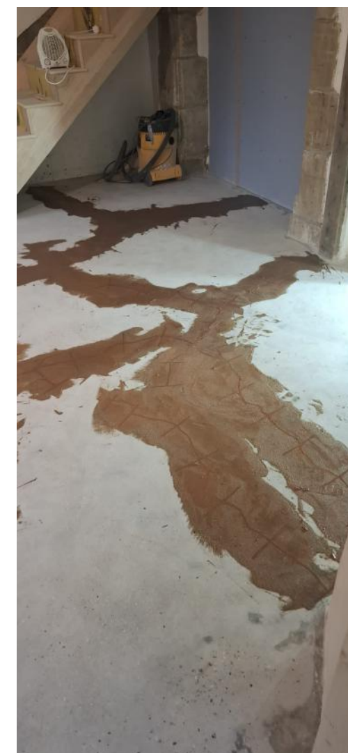
Living Room Interior: photographs show the modern blockwork wall and cracked rough concrete floor prior to the commencement of repairs/works were carried out.
