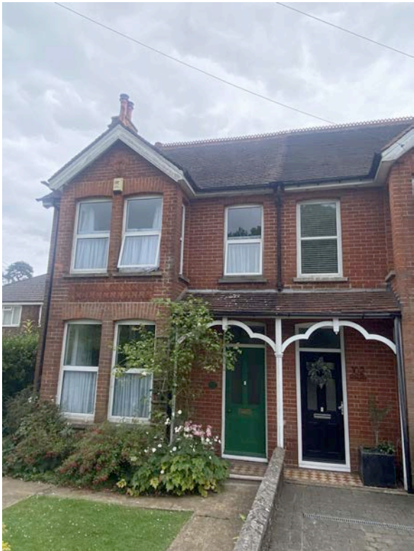
Front 104 & 102 Junction Rd Photograph
