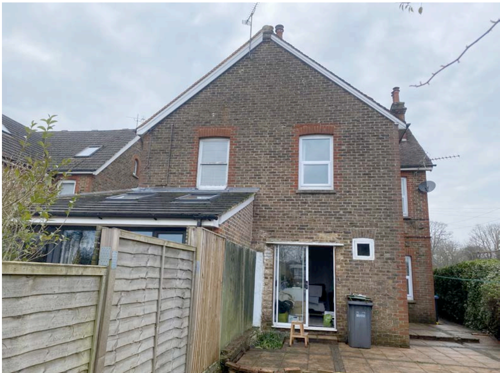
Rear 104 & 102 Junction Rd photograph
