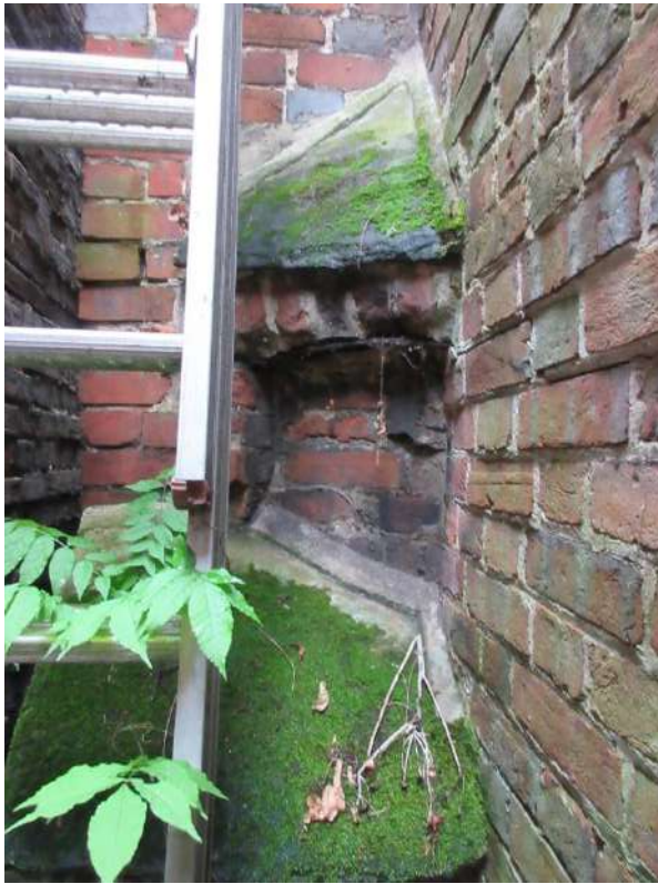
Figure 24 (left): Historic bread oven attached to the side (south) elevation of Somners.
