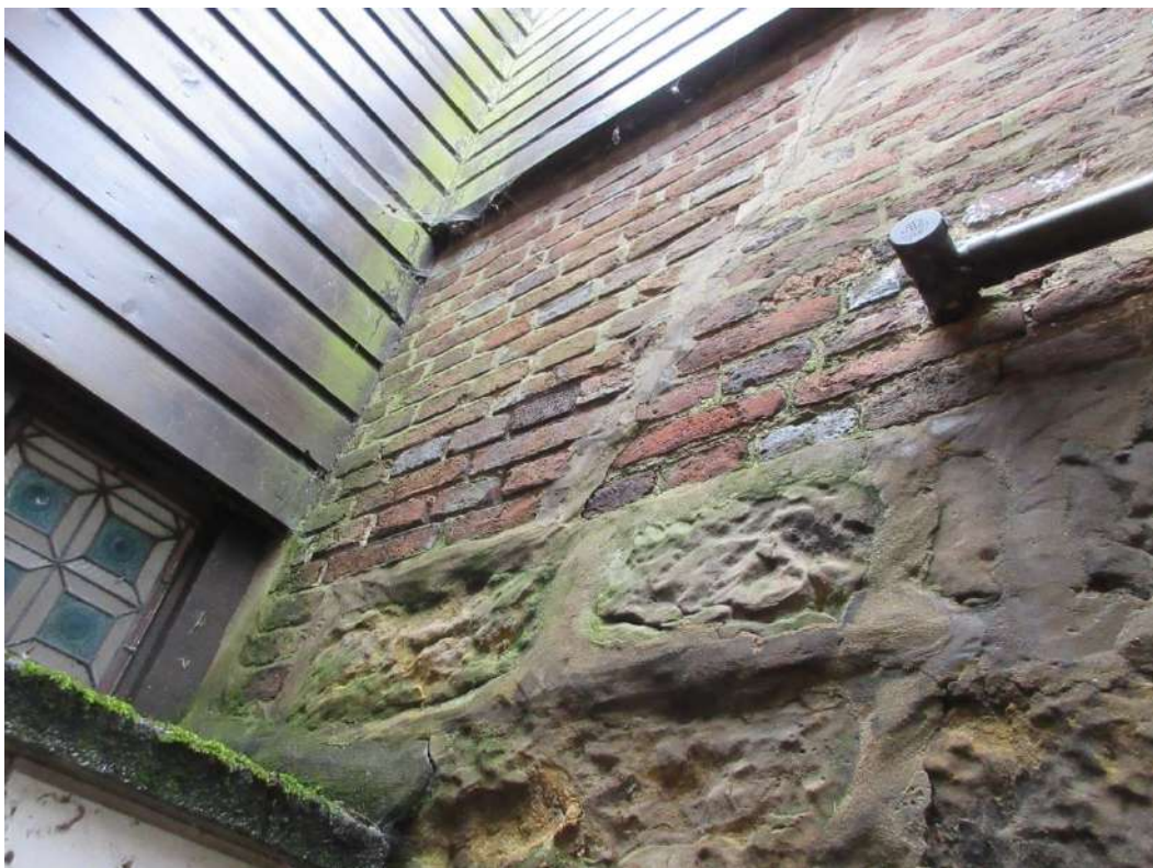
Figure 31: Side (north) elevation of The Friary in the gap between Somners and The Friary. Note modern timber boarding (to the modern two-storey extension on the left), and historic brickwork and stonework (on the right).
