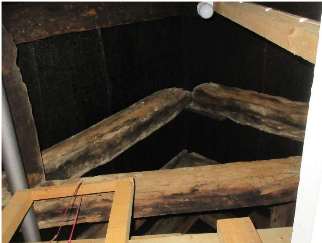
Figure 62: Interior of The Friary (roof space). Note original roof timbers (which are blackened).
