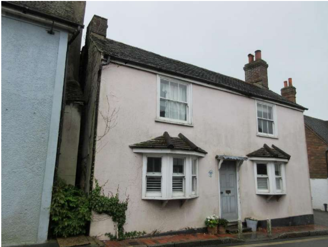
Figure 30: The Friary (Grade II).
