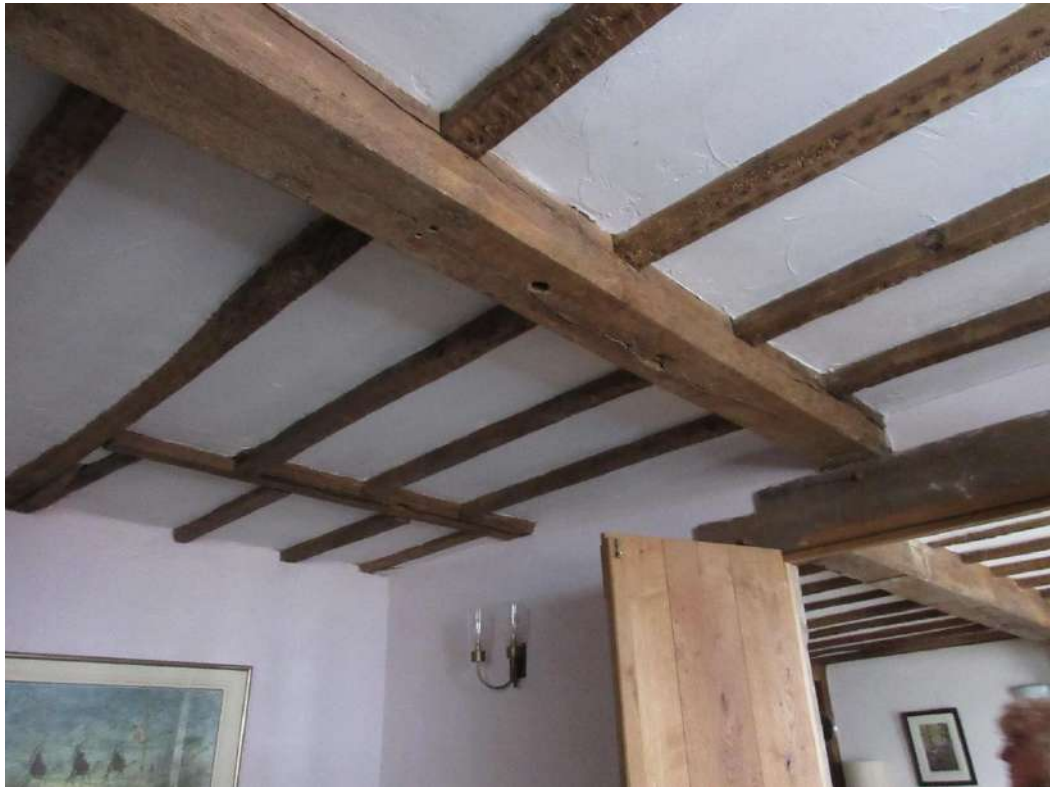
Figure 42: Interior of Somners (ground floor) – Ceiling timbers to room to the north, which do not align with those of the principal front room.
