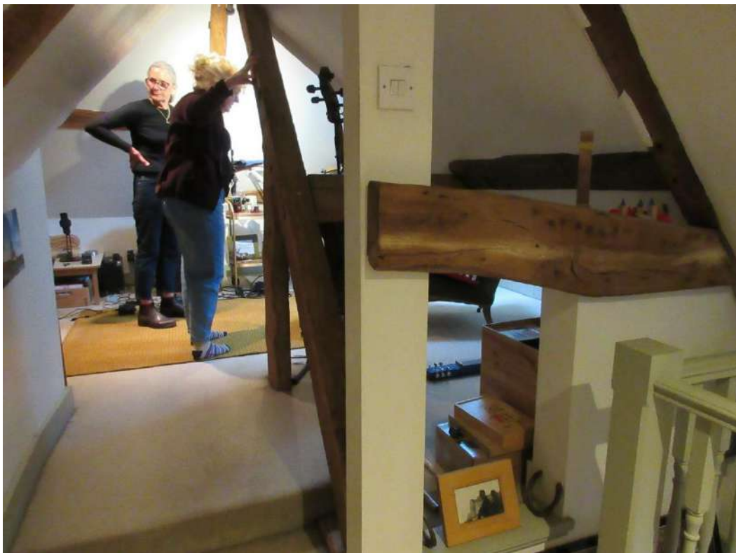
Figure 51: Interior of Somners (attic floor). Note original timber framing.
