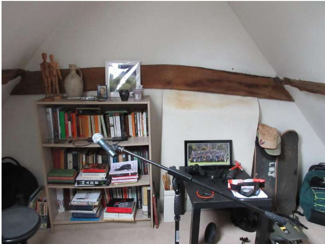
Figure 50: Interior of Somners (attic floor). Note original chimney breast and timber framing.
