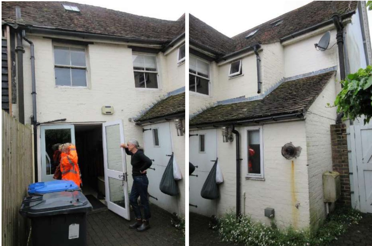
Figure 28 (left): Side (north) elevation of the rear extension to Somners (Grade II).
