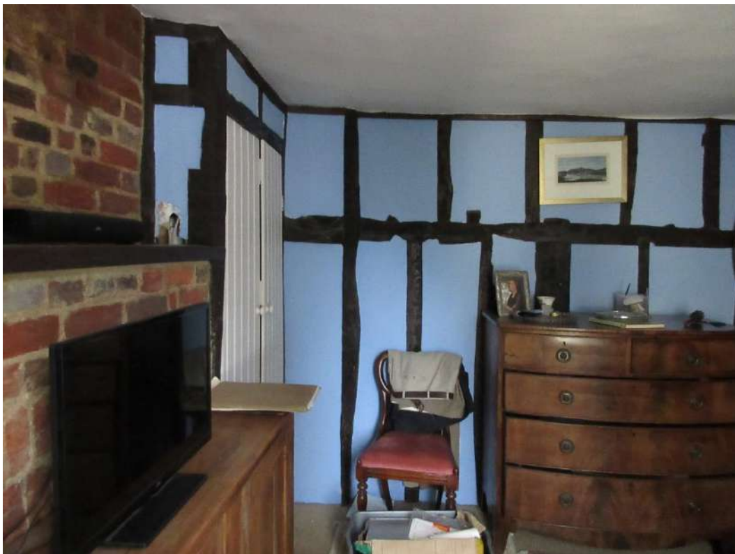
Figure 60: Interior of The Friary (first floor) – Front north bedroom. Note original timber framing, and historic fireplace.
