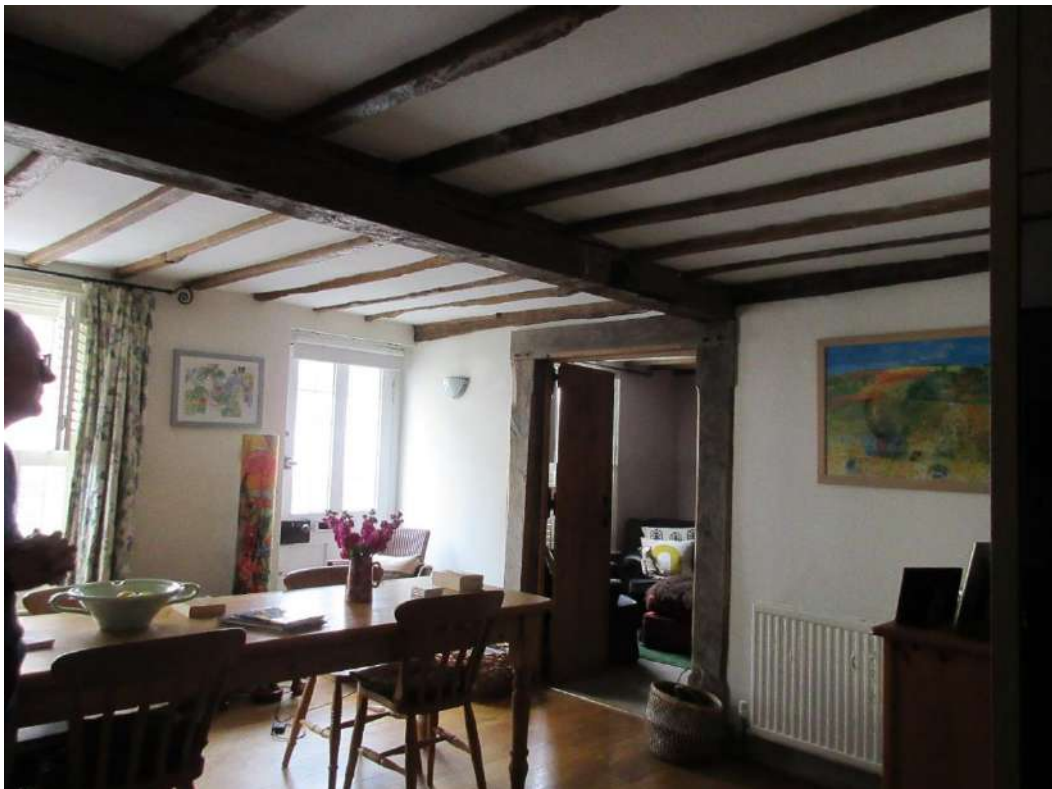
Figure 41: Interior of Somners (ground floor) – Front principal room. Note original ceiling beams, and unusually large door opening to the north.
