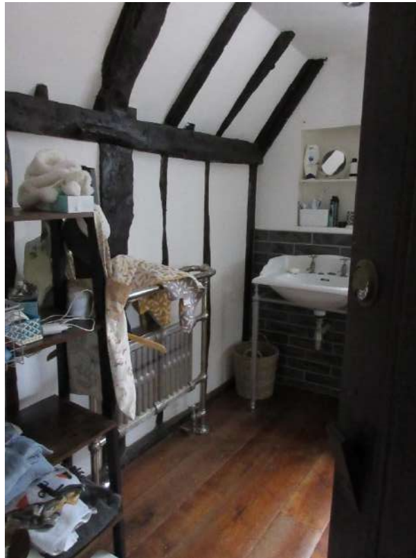
Figure 57: Interior of The Friary (first floor) – Room to the north. Note original timber framing.
