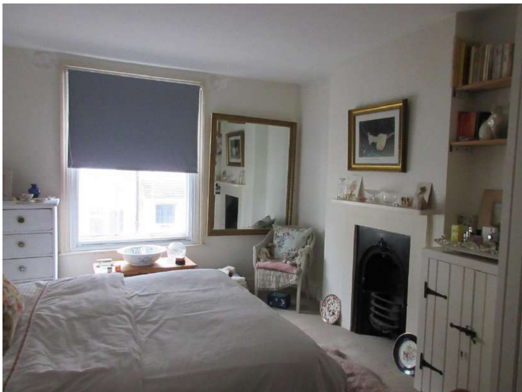
Figure 49: Interior of Somners (first floor) – Front bedroom. Note chimney breast, and Victorian sash windows.
