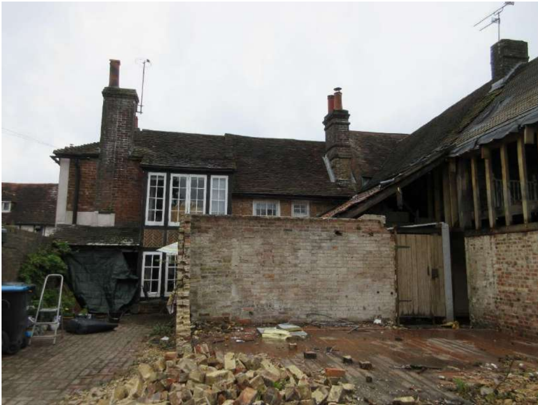
Figure 34: Rear (east) elevation of The Friary (Grade II).
