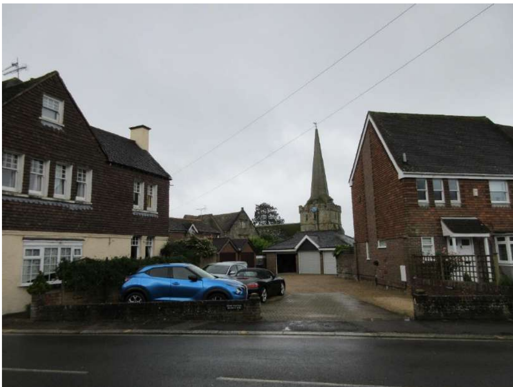
Figure 70: Southward view from South Street in the direction of the rear garden of the Site – with the spire of the Holy Trinity Church (Grade I) straight ahead. On the left is The Shades, and a glimpse of Cuckfield Church of England Primary School (Grade II); and on the right is Rosemary Cottage.
