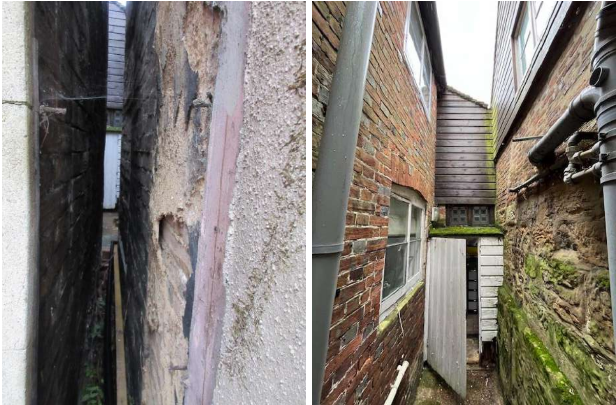
Figure 32 (left): Eastward view of the gap between Somners and The Friary, seen from South Street. Note historic render to north elevation of the western part of The Friary.
