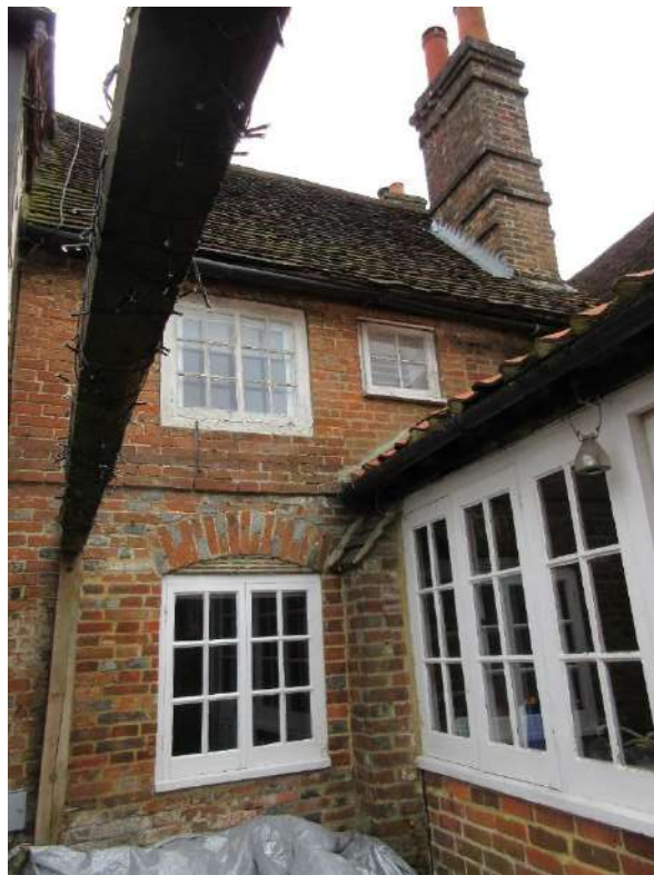
Figure 37: Part of rear (east) elevation of The Friary (Grade II), and part of the modern single-storey rear extension.
