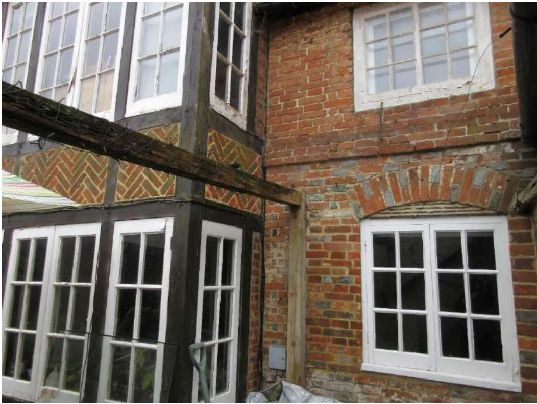
Figure 38: Rear (east) elevation of The Friary (Grade II).
