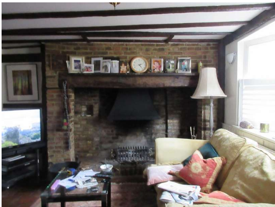
Figure 52: Interior of The Friary (ground floor) – South part of front principal room. Note original fireplace, and timber framing.
