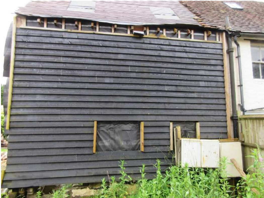
Figure 21: Side (north) elevation of reconstructed rear extension to Somners (Grade II).
