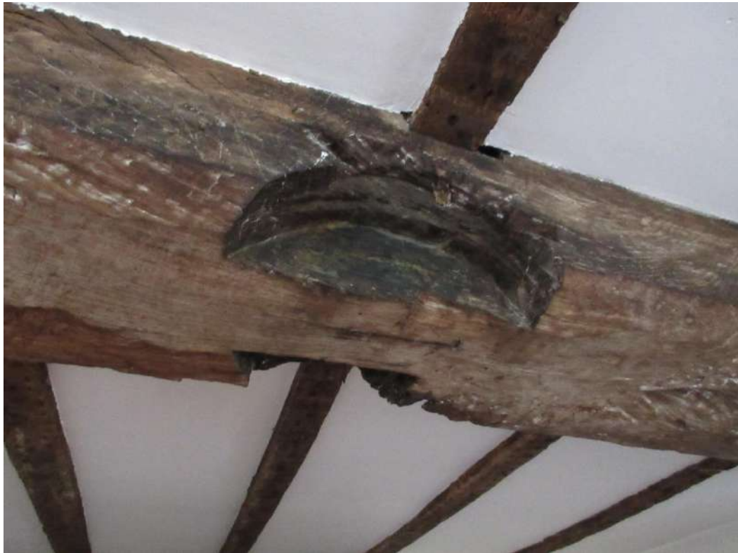
Figure 48: Interior of Somners (first floor) – Room to the rear (east). Note original timber framing, together with an indentation which provides an insight into the former use of the room as a workshop.
