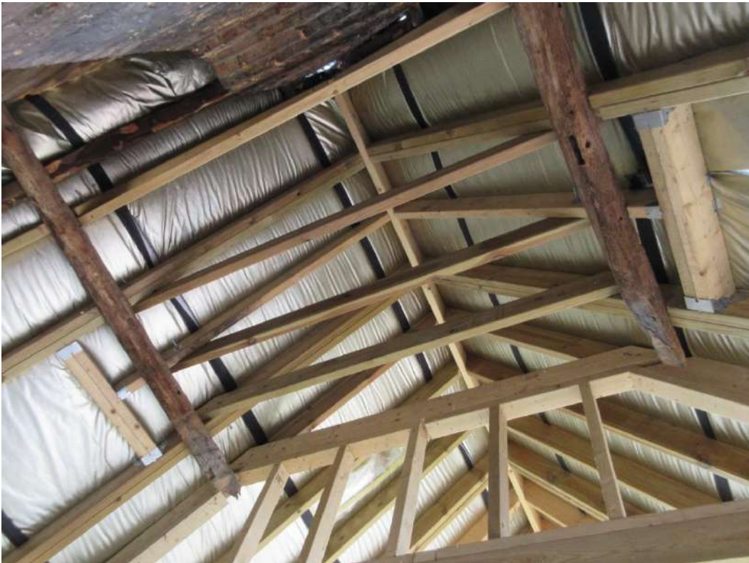
Figure 20: Reconstructed roof timbers of rear part of Somners (re-using two historic timebers).
