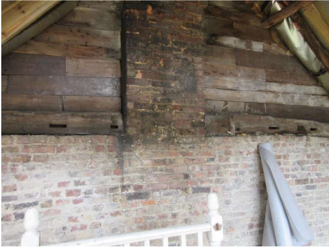
Figure 19: Interior of east elevation of rear part of Somners.
