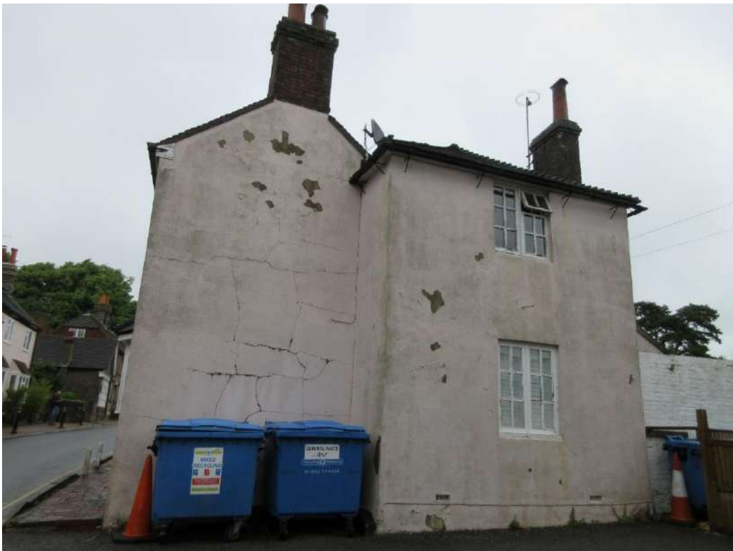
Figure 39: The side (south) elevation of The Friary (Grade II).
