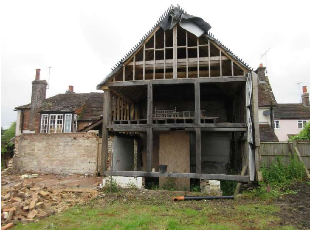
Figure 4: Rear (east) elevations of The Friary (Grade II) and Somners (Grade II), in May 2024, once the works for the consented scheme had commenced.
