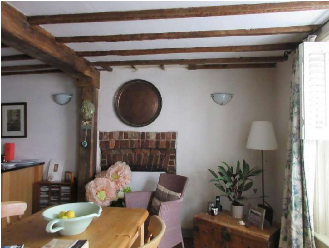
Figure 44: Interior of Somners (ground floor) – Front principal room. Note chimney breast and original timber framing.
