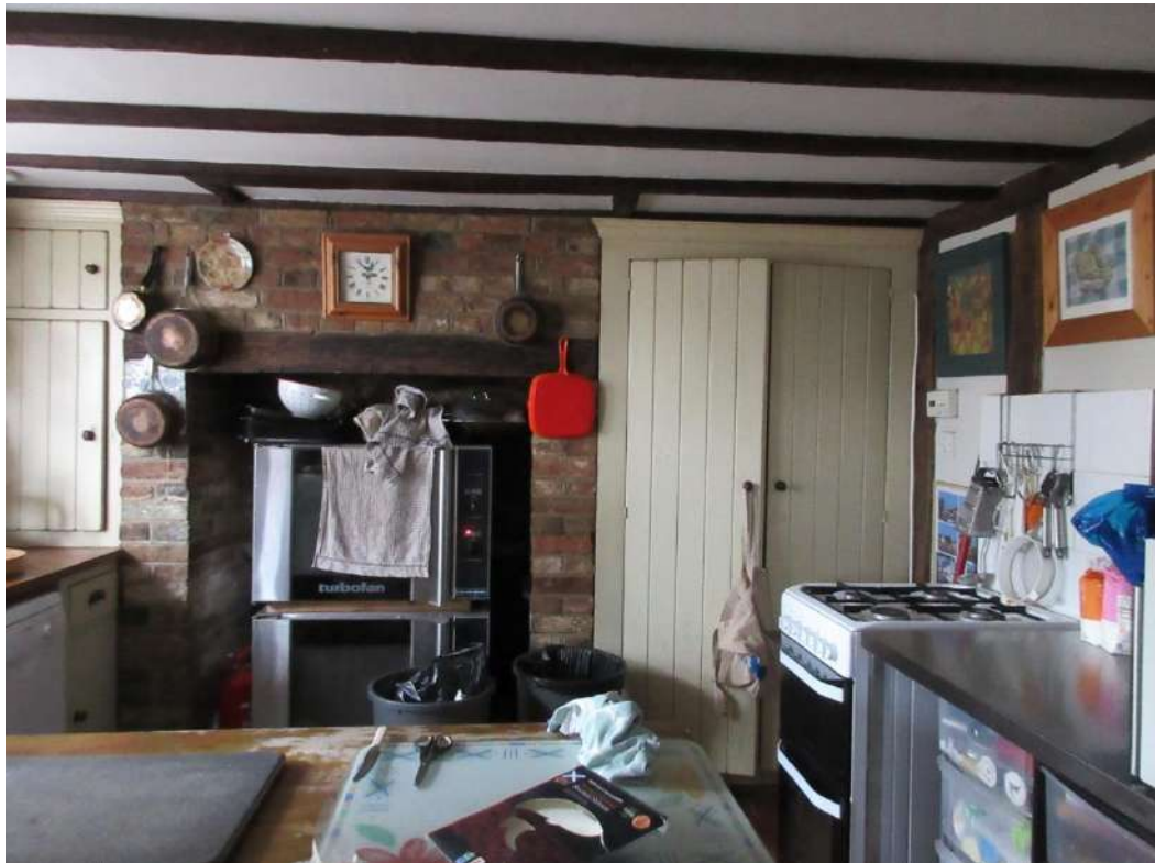
Figure 53: Interior of The Friary (ground floor) – North part of front principal room. Note fireplace, and original timber framing.
