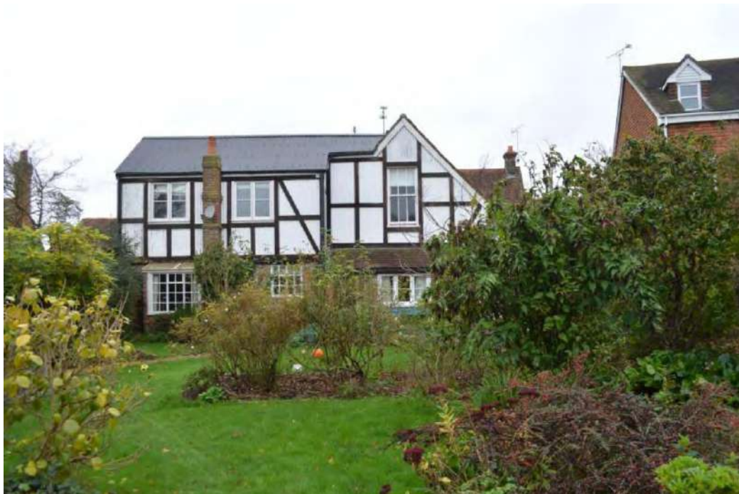
Figure 3: Rear (east) elevations of The Friary (Grade II), Dumbrells, and Somners (Grade II), prior to enactment of application DM/18/3863.
