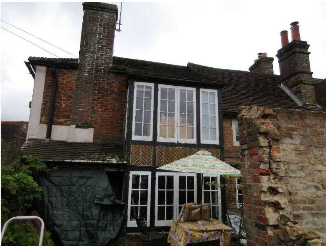
Figure 35: Rear (east) elevation of The Friary (Grade II).
