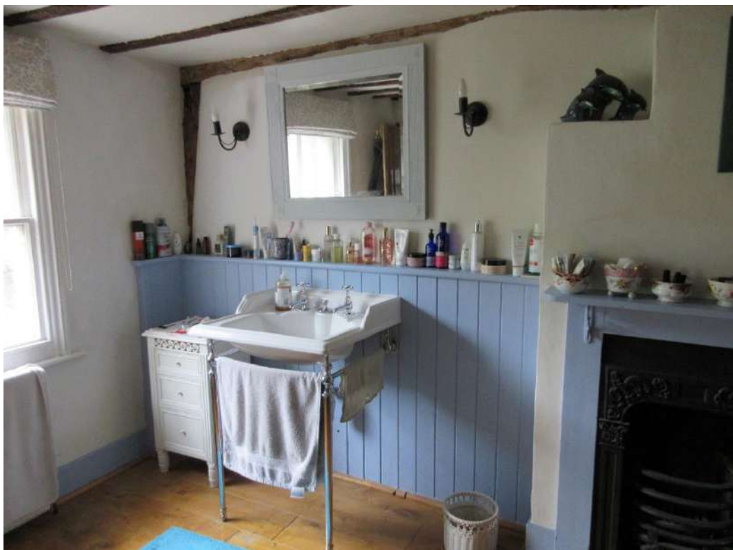
Figure 47: Interior of Somners (first floor) – Room to the rear (east). Note original timber framing, and Victorian chimney breast and fireplace. (The proposals involve the provision of a new door opening to the left of the chimney breast.)
