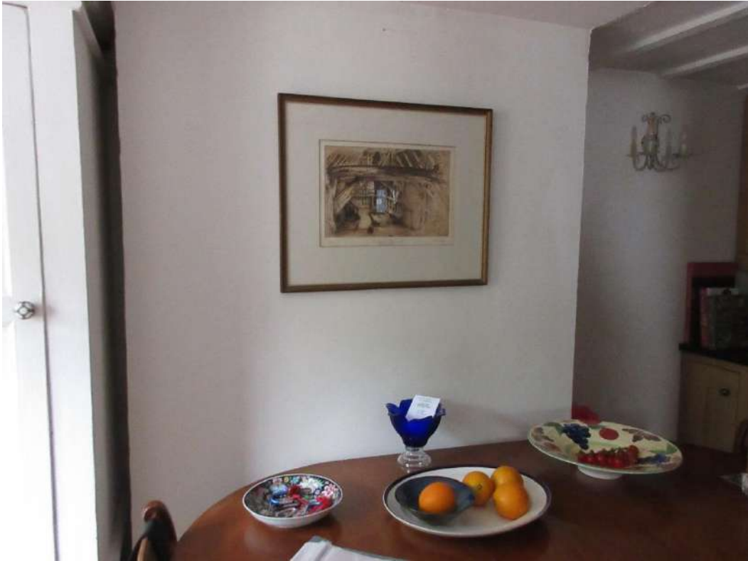
Figure 40: Interior of Somners (ground floor). Note Victorian chimney breast to the rear (east) wall. (The proposals involve the provision of a new door opening to the left of the chimney breast.)
