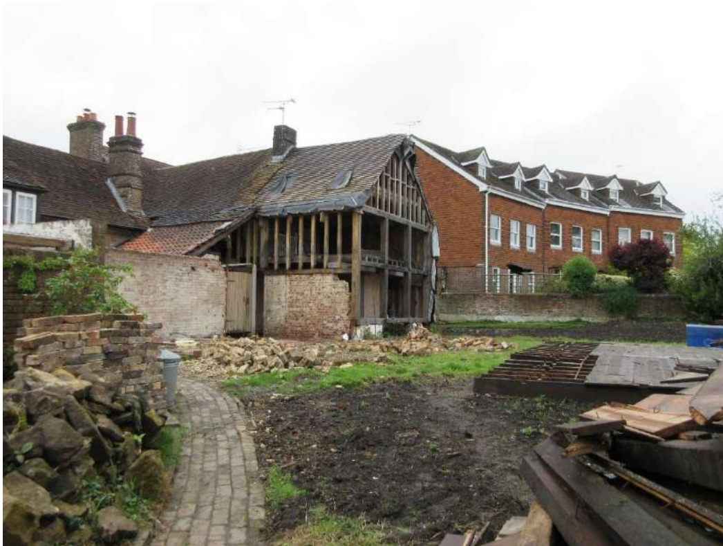
Figure 6: Northward view across rear garden of Site.
