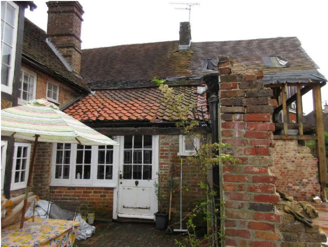
Figure 36: Side (south) elevation of the modern single-storey rear extension to The Friary (Grade II). Note modern mono-pitched pantiled roof which continues from the pitched roof of Somners (creating a “cat-slide” roof effect).
