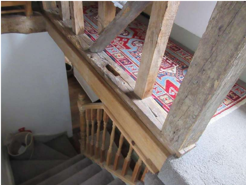
Figure 45: Interior of Somners (stairs between ground and first floors). Note modern balustrading, and timber framing at first floor level.
