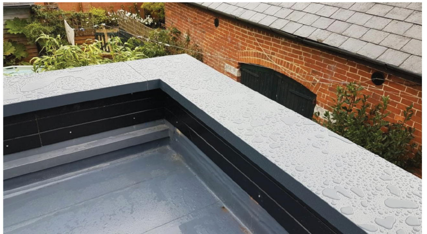
Fig. 2. GRP roof finish with aluminium coping.
