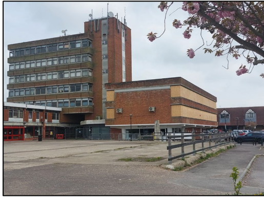
Figure 1: Boarded up building
