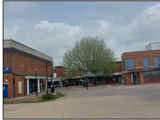
Figure 2: Central courtyard with boarded up buildings
