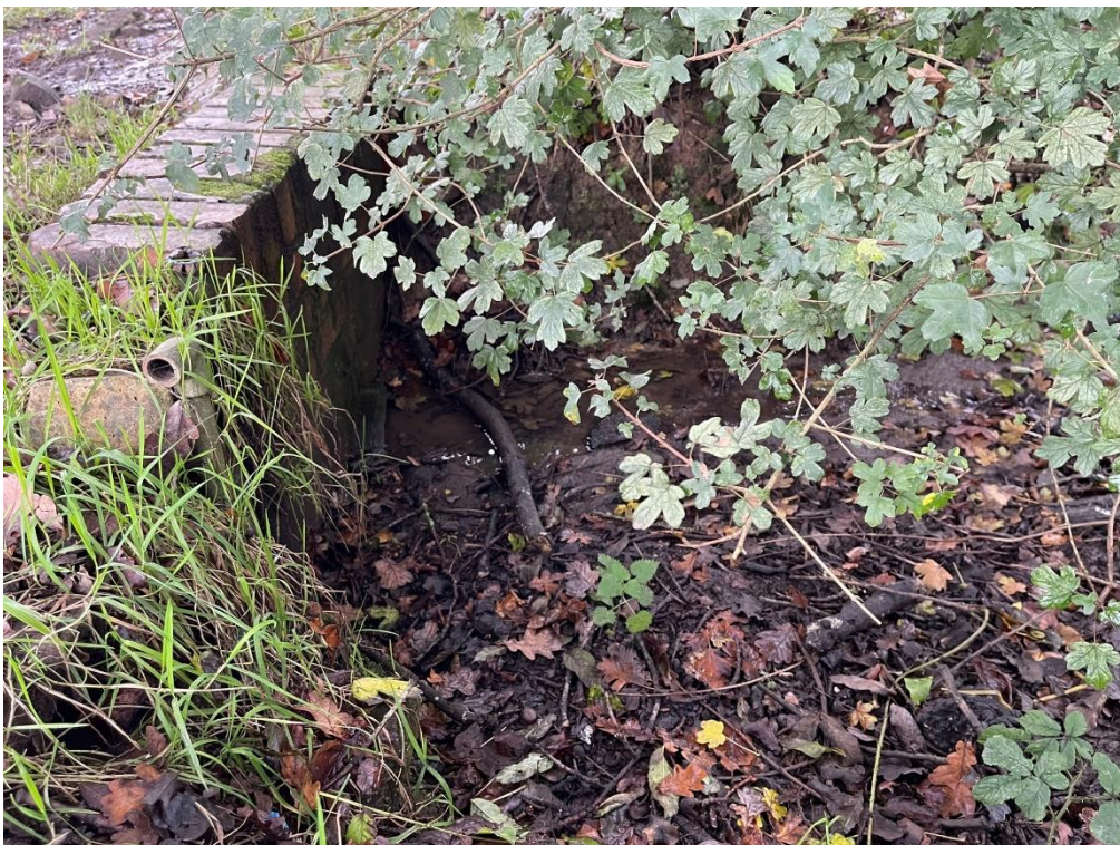
Image 02 – Showing the wet ditch to the eastern boundary of the client's agricultural field, which the new clean effluent and the attenuated controlled stormwater flows are to discharge to
