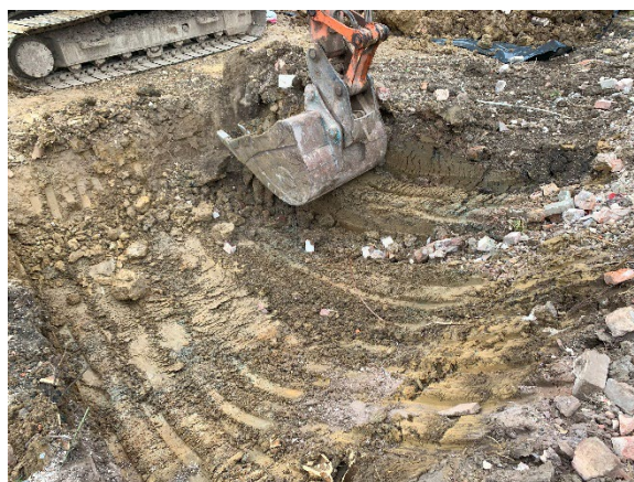
Plate 2. Early stages of excavation works.
