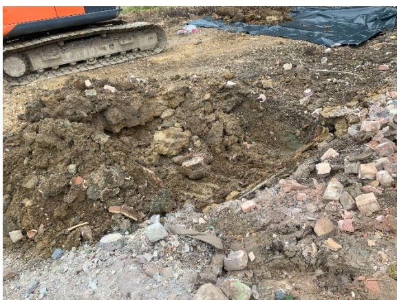
Plate 1. Early stages of excavation works.
