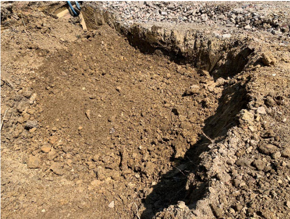
Plate 5. Low reading arisings backfilled into the trial pit.
